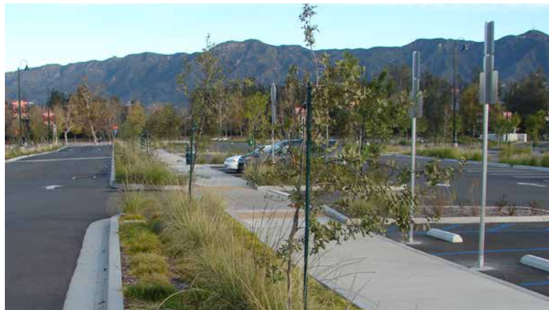
The LA Zoo parking lot improvement project removes trash and other pollutants in urban runoff using bioretention cells, permeable pavement, and drought tolerant plants.
