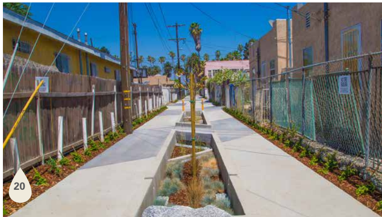
The Avalon Green Alley North is a collaborative effort to green a network of alley segments within residential neighborhoods of Los Angeles.
