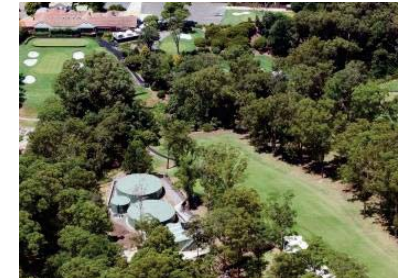
Golf course facility (irrigation)
