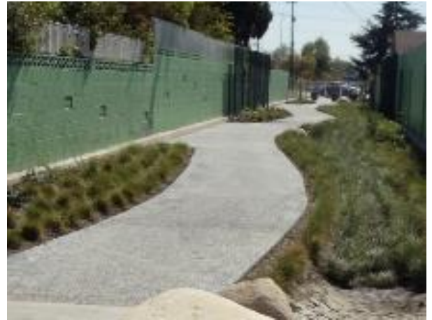
Elmer Paseo is one the City's "Green Alley" projects, capturing stormwater for infiltration and recharge of groundwater.
