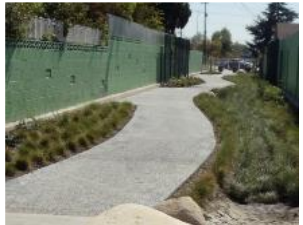
Elmer Paseo is one the City's "Green Alley" projects, capturing stormwater for infiltration and recharge of groundwater.
