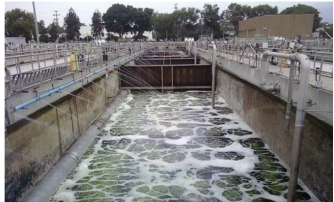
To increase water recycling at LAGWRP key modifications are in the planning stage such as providing additional equalization capacity.
