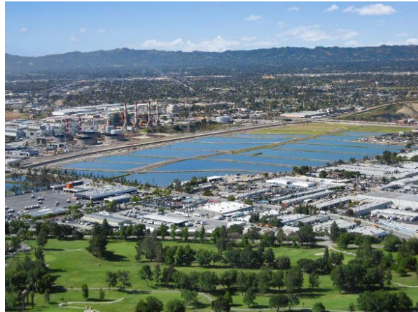
The Groundwater Replenishment Project will recharge up to 30,000 acre-feet of purified recycled water per year into the San Fernando groundwater basin at the Hansen Spreading Grounds (shown) and Pacoima Spreading Grounds for percolation.
