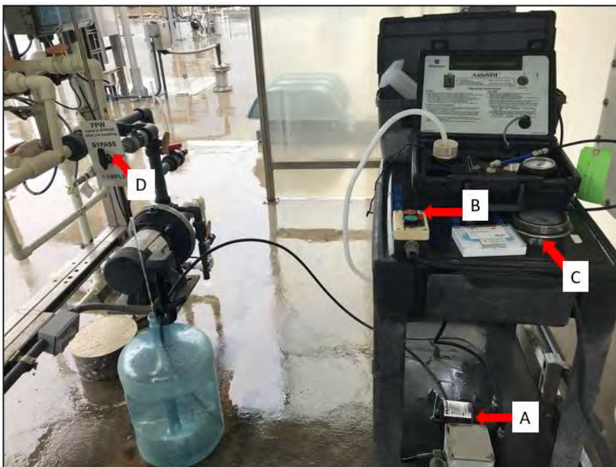
AutoSDI unit set up for readings at FPW on GWRS campus. At this location source water is less than 30psi so an auxiliary pump system is used. Note the source water is delivered from the storage container into the auxiliary pump unit and into the AutoSDI unit using black tubing. (A) Auxiliary pump unit (B) auxiliary pump control (C) pressure gauge from auxiliary pump (D) FPW source water valve.
