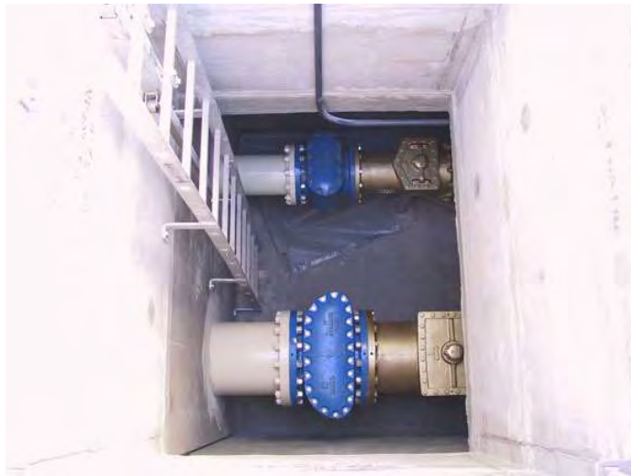
View down into meter vault.
