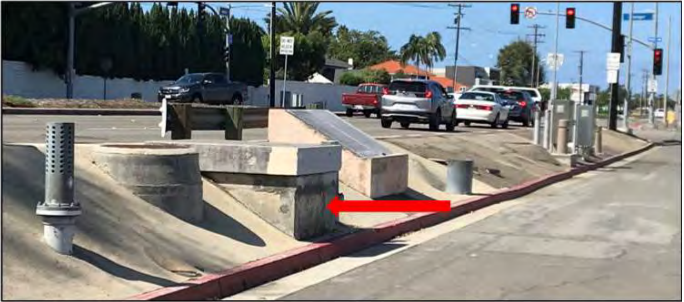
Figure 12 Looking west along Adams Avenue. The OC-44 flow meter vault in the foreground, the City of Huntington Beach distribution system connection can be seen in the background. The red arrow indicates access into the vault.
