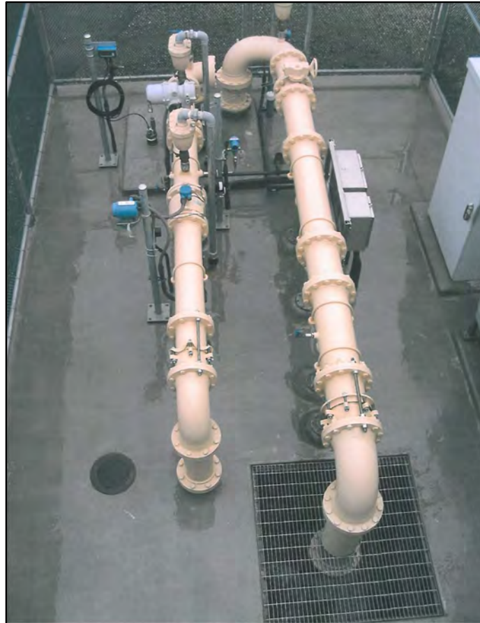
Figure 7 Modern Well I-36. I-36 is a single casing Modern Well that injects into the merge zone between the Talbert and Lambda aquifers. I-36 is located along the west levee of the Santa Ana River at Adams Ave.
