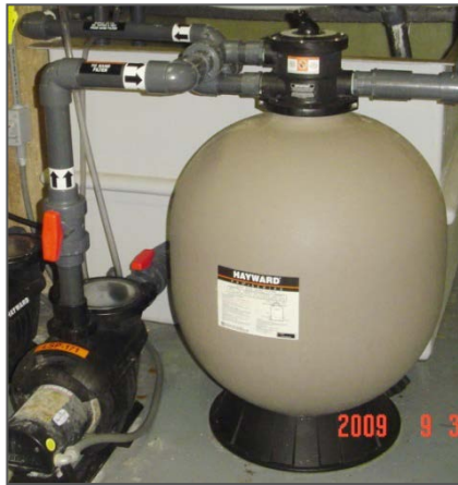
Figure 7.66 - Typical Sand Filter
