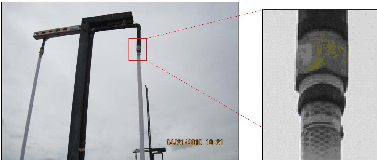
Flow control valves installed on hoses
