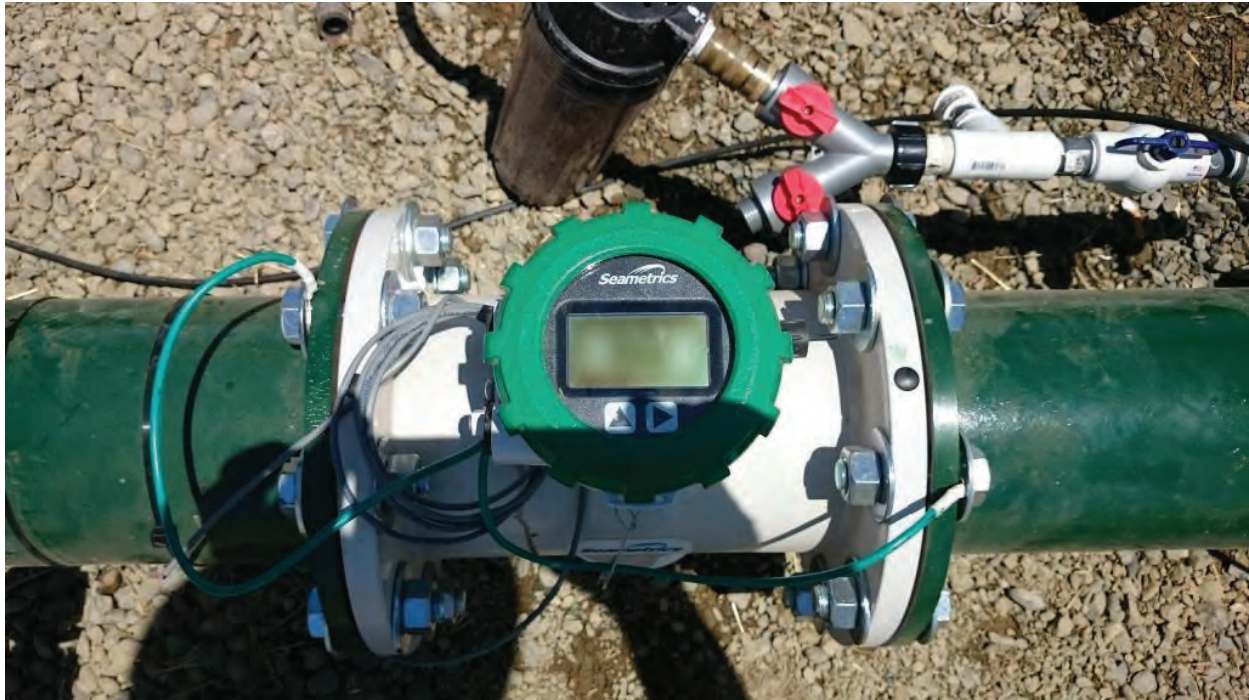
Figure 2-14. Flow Meter, Sampling Ports, and Bio-Indicators Sample Filter
