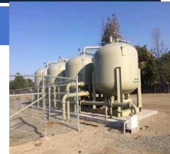
1,2,3-TCP Wellhead Treatment
