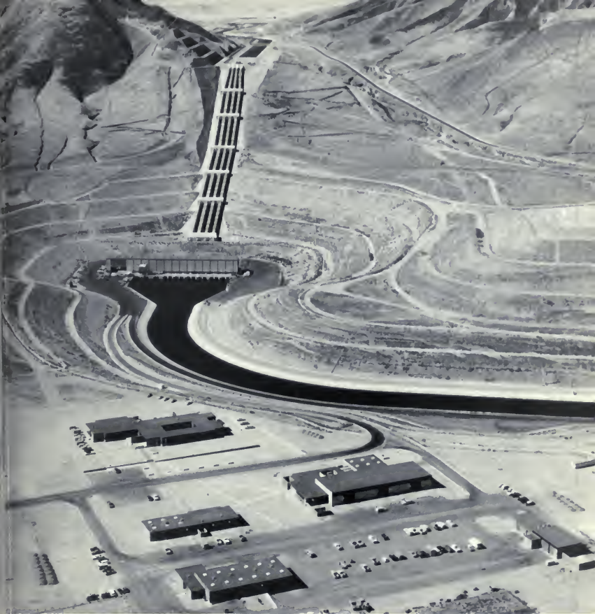
Figure 22 WIND GAP PUMPING PLANT AND SAN JOAQUIN OPERATIONS AND MAINTENANCE CENTER
