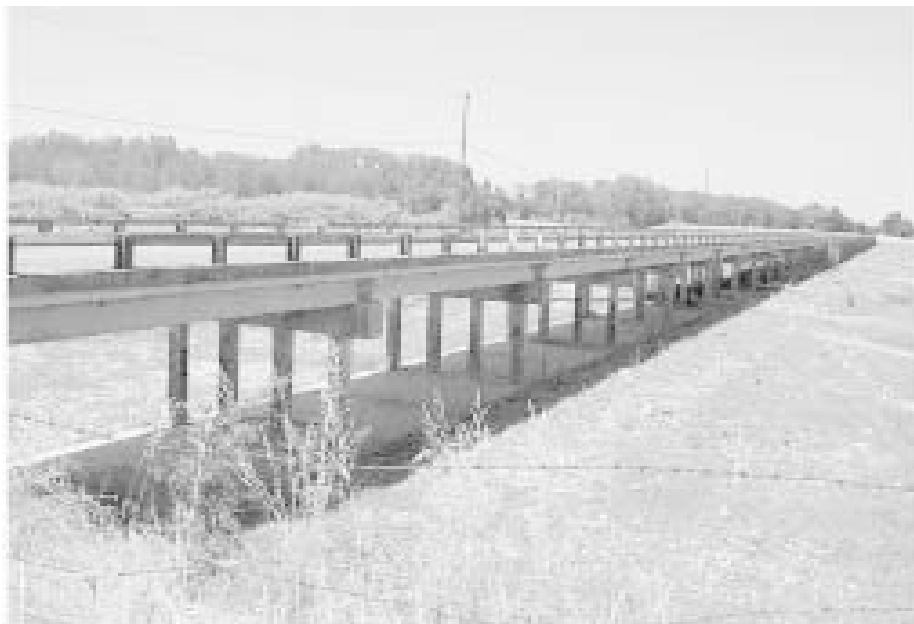
Tisdale Weir (Photo by: Flood Operations Center Archive)
