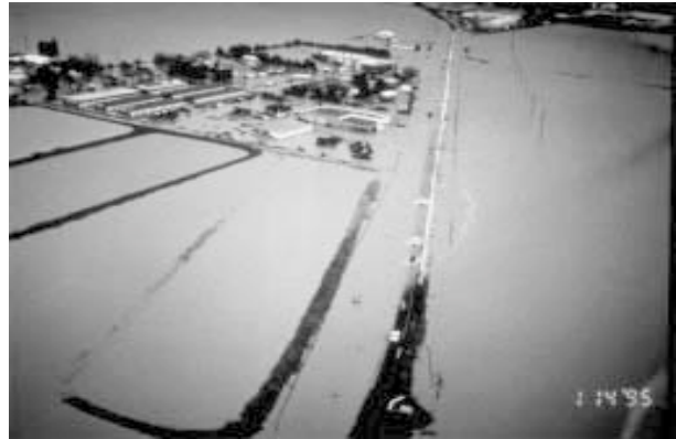
Aerial view toward the northeast of flooded areas covering Highway 20 and the southwestern section of the town of Colusa (photo taken January 14, 1995/Rick Burnett, DWR Flood Flight Specialist).
