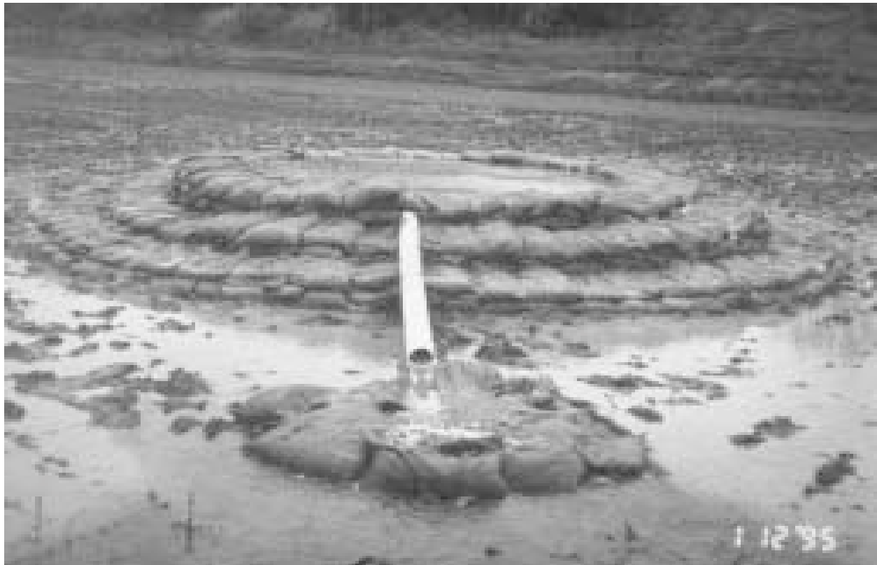
Above: Sack ring constructed to reduce the flow and prevent further discharge of earthen material from a boil that developed near Elk Slough on Merritt Island (RD 150). Below: Levee repairs on Webb Tract (Reclamation District 2026) funded by the SB 34 Special Flood Control Projects Program.
