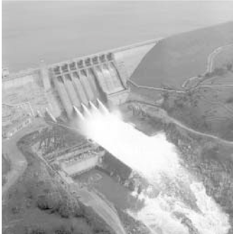
Flood control releases from Folsom Dam to the American River reached 50,000 cubic feet per second in March.
