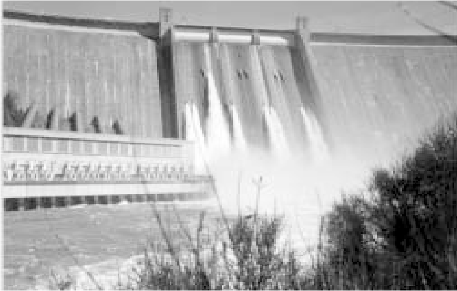
Flood control releases from Shasta Dam to the Sacramento River reached 79,000 cubic feet per second in March.
