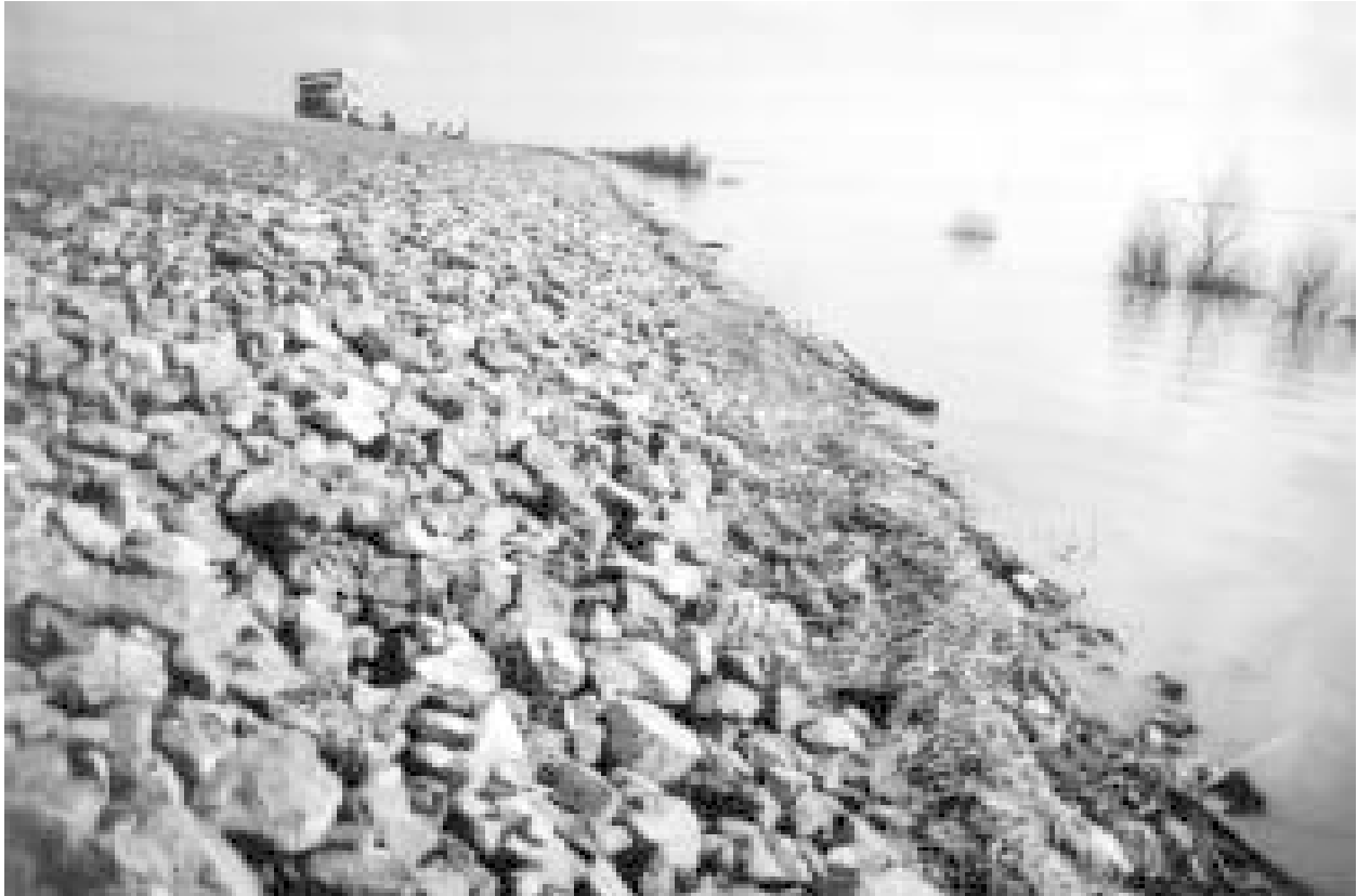
The photographs above and below show wave wash protection repairs in Reclamation District 108 along the Colusa Basin Drain.
