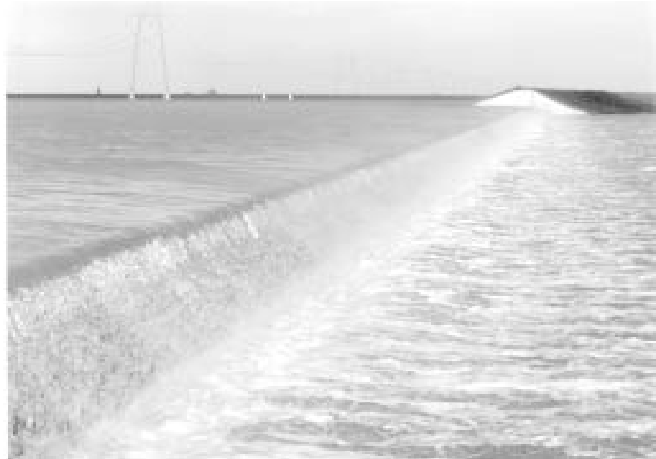
Cache Creek Settling Basin overflows in 1995.
