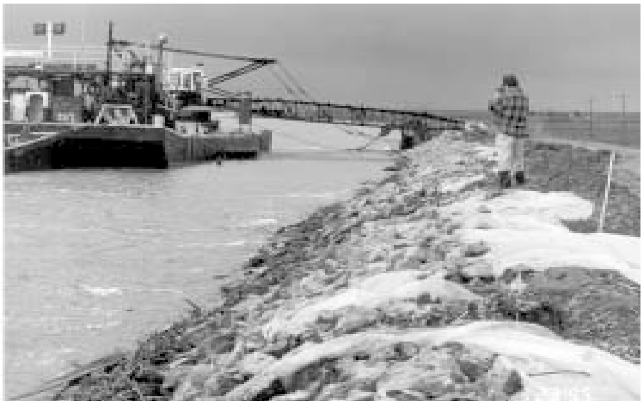
Above: Sack ring constructed to reduce the flow and prevent further discharge of earthen material from a boil that developed near Elk Slough on Merritt Island (RD 150). Below: Levee repairs on Webb Tract (Reclamation District 2026) funded by the SB 34 Special Flood Control Projects Program.
