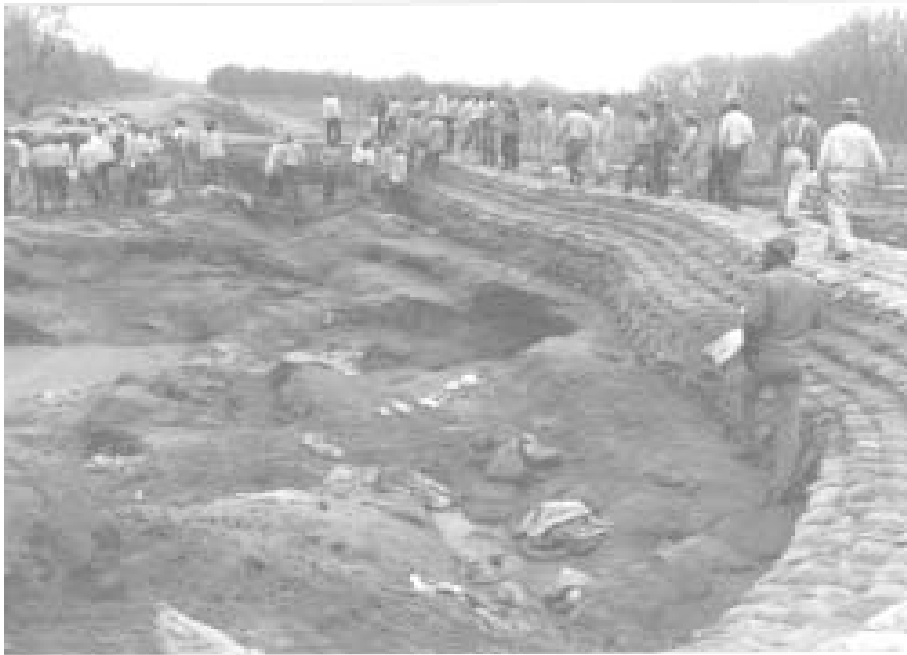
These photos show the 43,000 sandbag structure constructed to close breach in the Deseret Levee in Butte County. Below is an aerial view of the completed structure.
