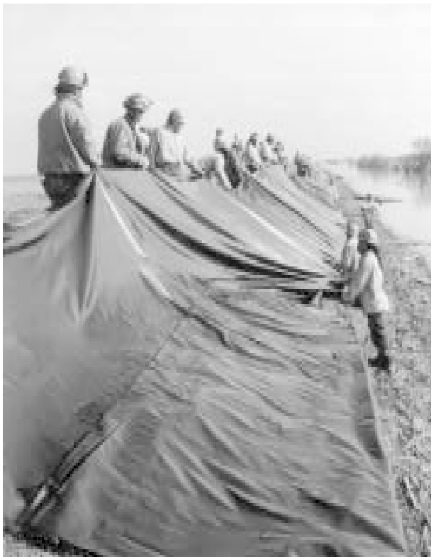
The photographs above and below show wave wash protection repairs in Reclamation District 108 along the Colusa Basin Drain.
