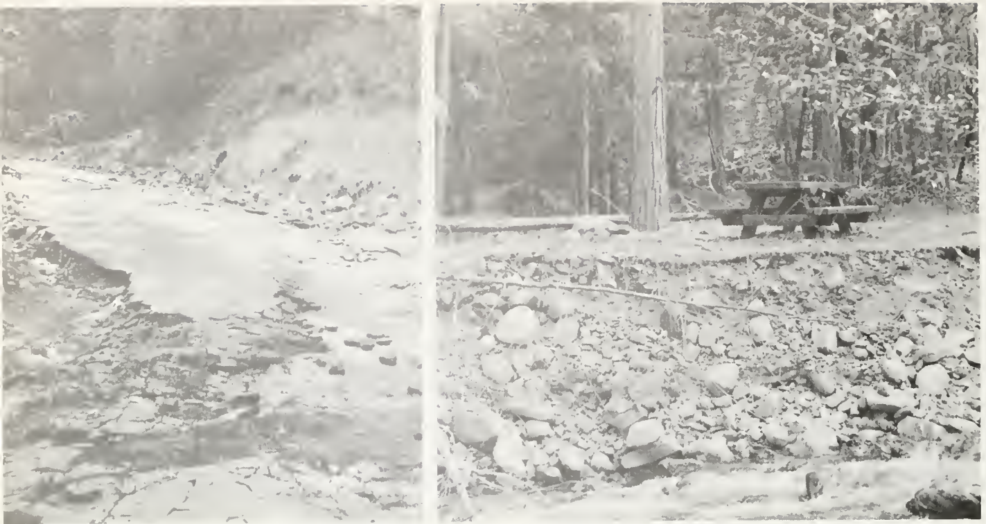
Damage caused by high water at O'Neil Creek campground in Klamath River basin: eroded paving in roadway (upper left), a washed out creek bank (upper right), and culverts and abutment exposed when the roadway was destroyed (below). (DWR Photos)
