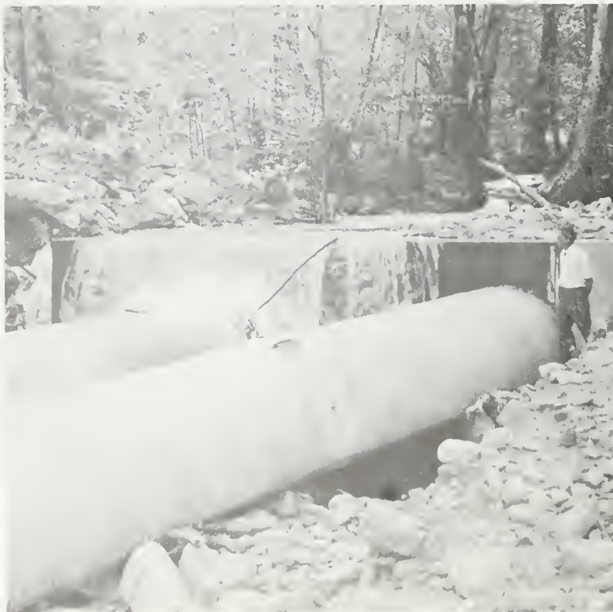
Damage caused by high water at O'Neil Creek campground in Klamath River basin: eroded paving in roadway (upper left), a washed out creek bank (upper right), and culverts and abutment exposed when the roadway was destroyed (below). (DWR Photos)
