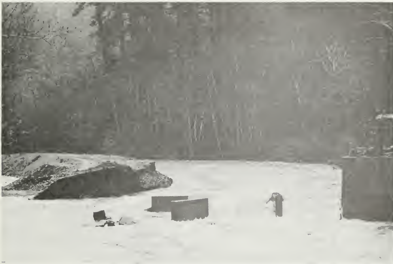
Washout at diversion dam on Last Man Creek at Humboldt County fish hatchery. (DWR Photo)
