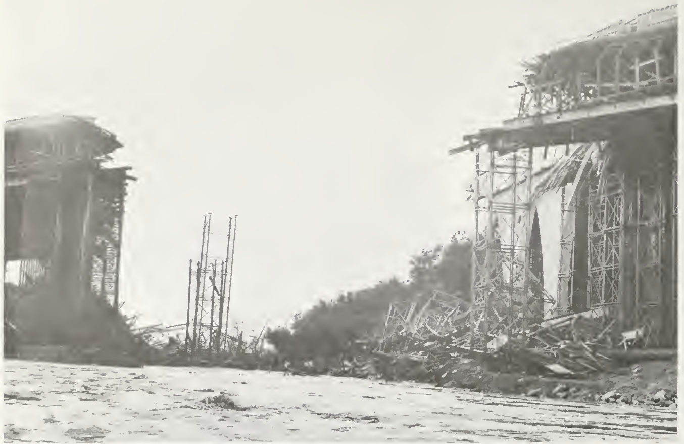
Above, Devil's Gate Reservoir filled and sent water over the spillway of the dam to Arroyo Seco. On February 11, 1973, the rushing water reclaimed the natural channel that had been occupied by the Foothill Freeway bridge falsework. (Photo by the Montrose Ledger)
