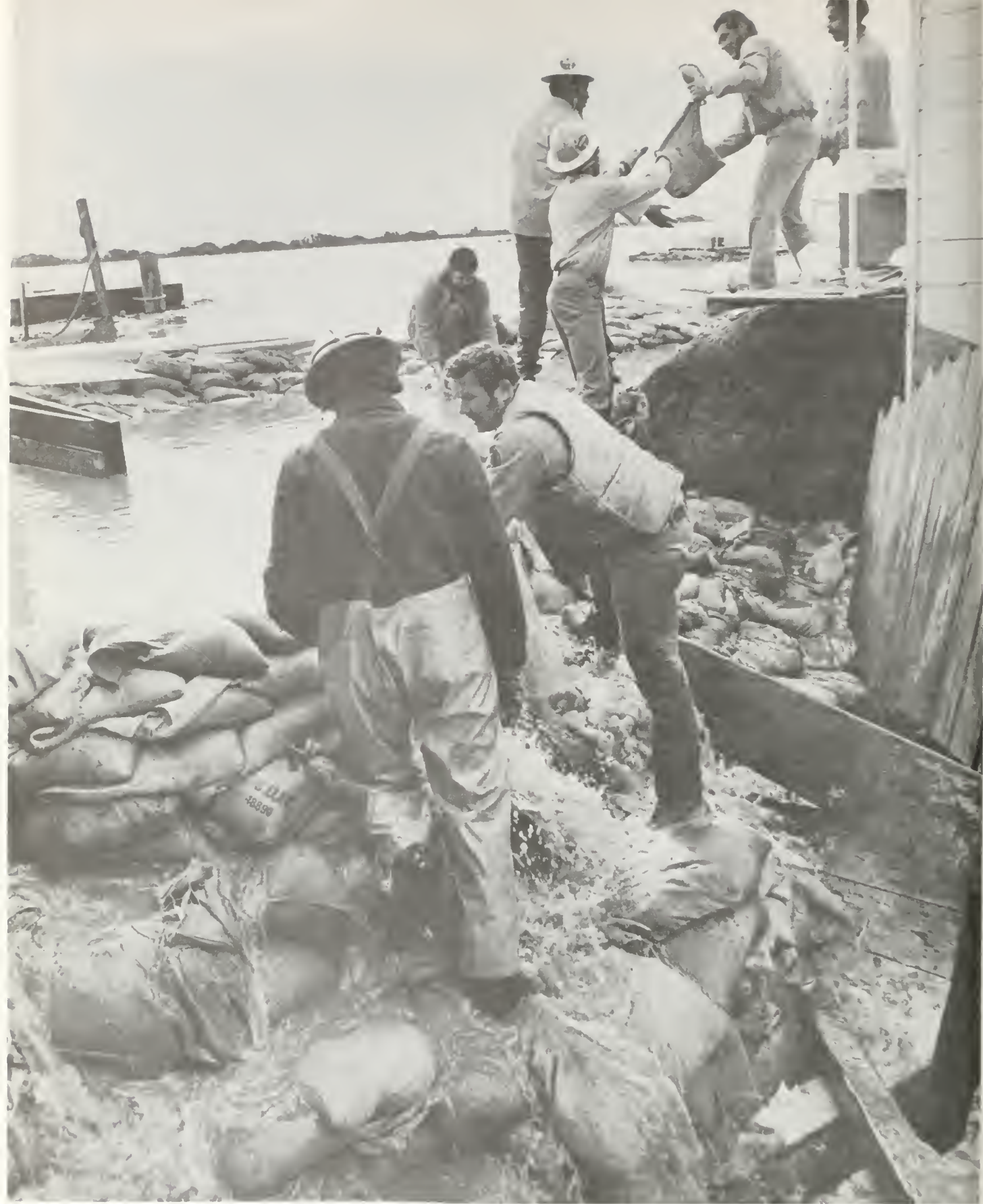
Flood fight operations during flooding of Edgerly Island in the Napa River delta on January 17, 1973. (Photo by the Napa Register)
