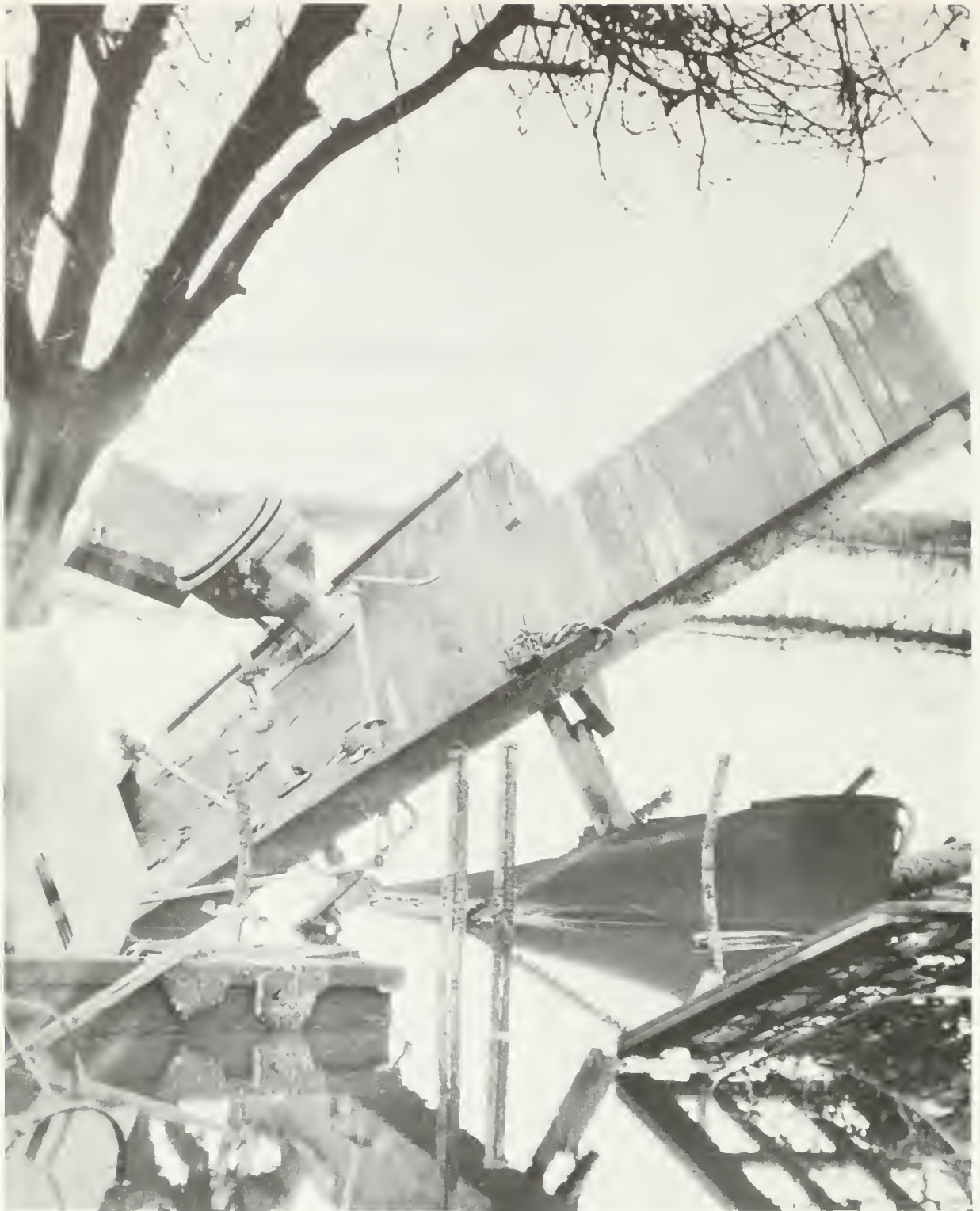
Remains of a flood-devastated home on Tyler Island Road three months after the Brannan-Andrus Islands levee break.
