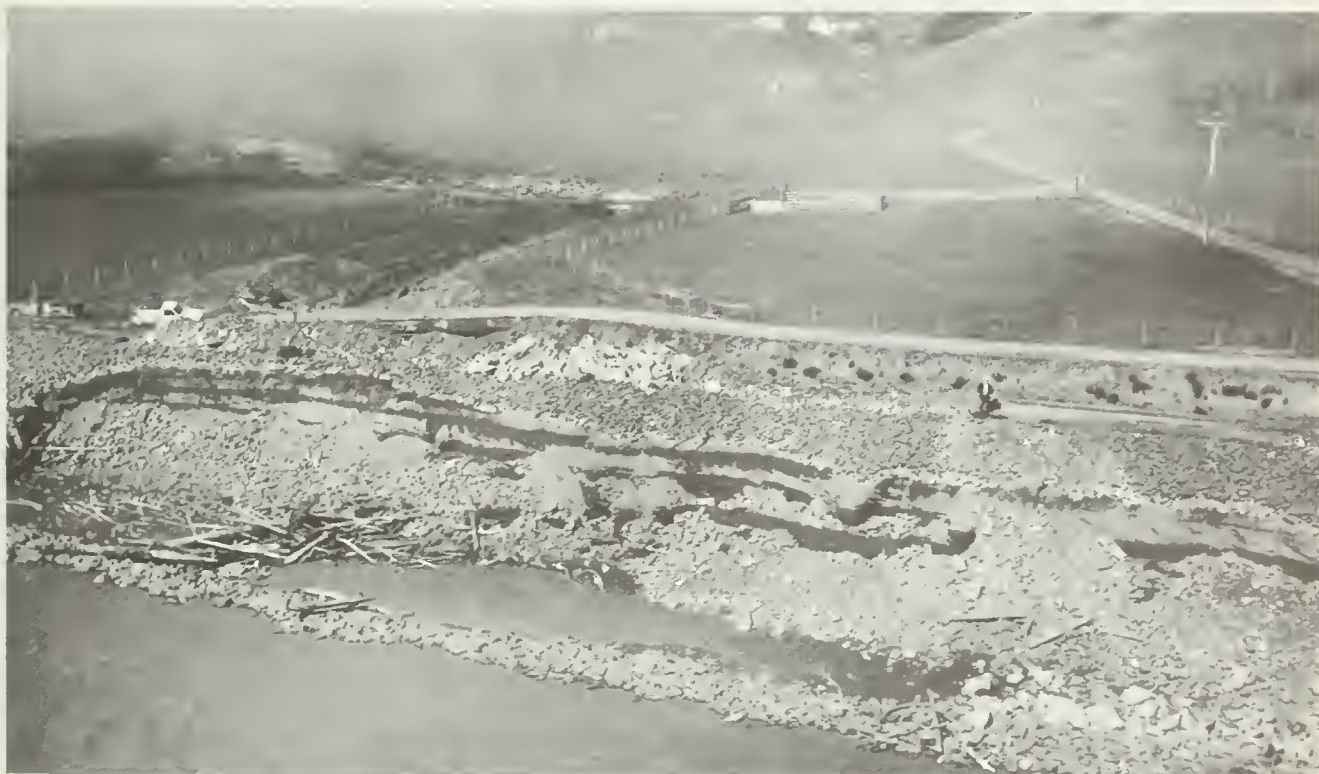
Levee erosion along Redwood Creek, Humboldt County, March 7, 1972.
