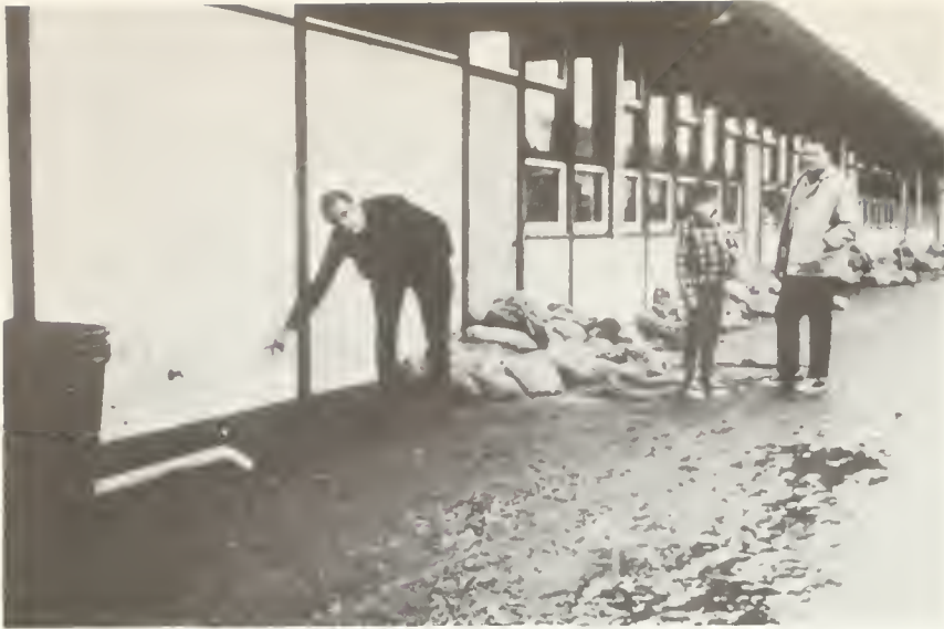
Carpinteria High School, Carpinteria, Santa Barbara County. Man is pointing to high-water mark left by flooding during December 1971.
