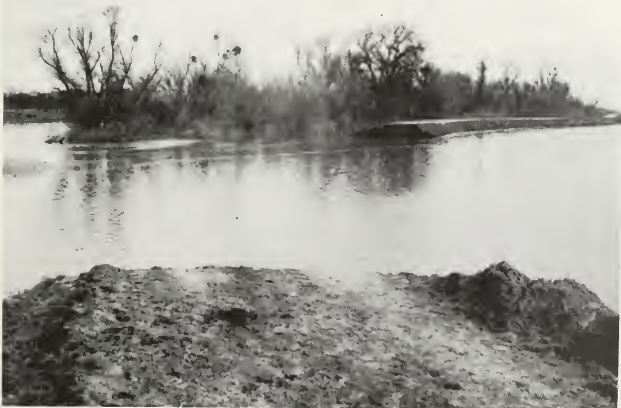
The left levee of the Stanislaus River, near the confluence of the San Joaquin River, was breached on January 27, causing inundation of an extended area of farm land.
