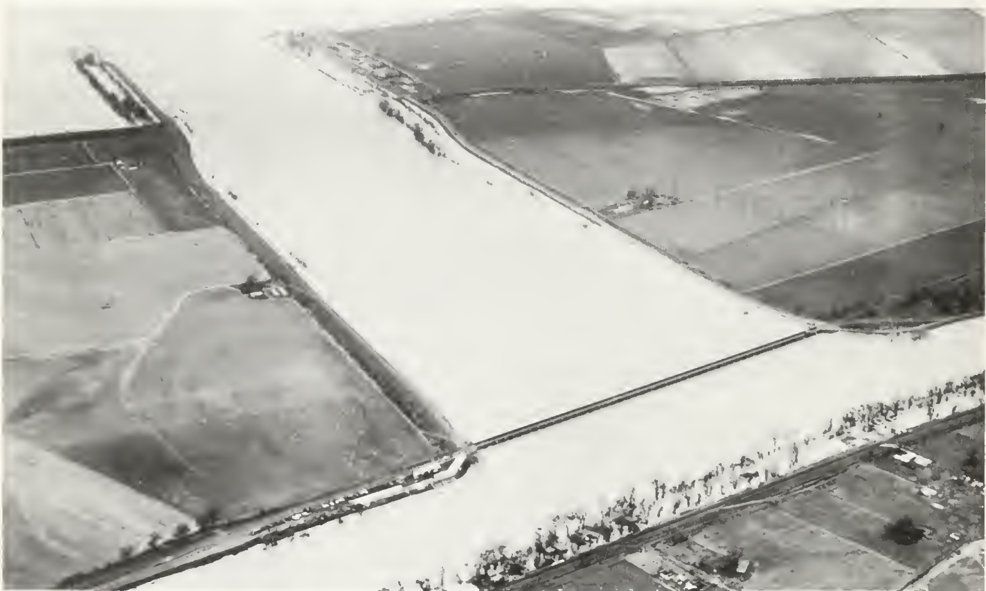
The Sacramento Weir diverts excess flows in the Sacramento River to the Yolo Bypass. Photograph - courtesy of Department of Water Resources Graphic Services.
