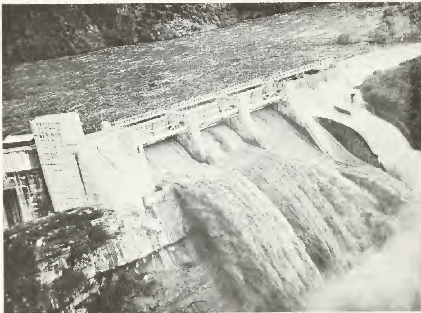
Gibraltar Dam on Santa Ynez River Photograph -courtesy of Santa Barbara County Flood Control and Water Conservation District.
