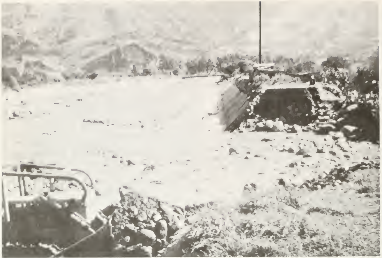
High flows in Southern California streams destroyed levees and bridges.
