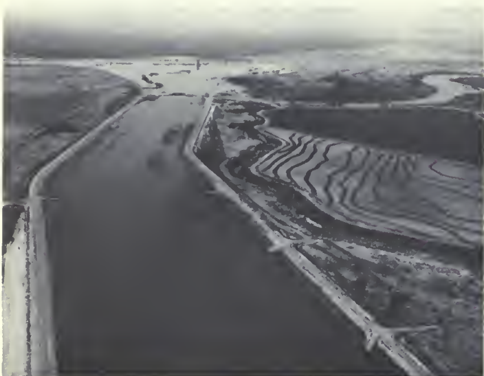
Snowmelt runoff in the San Joaquin River being diverted into the Chowchilla Canal Bypass.
