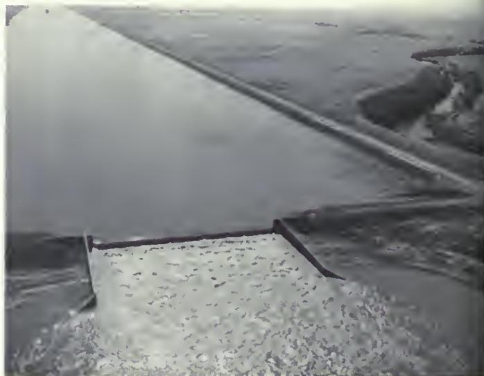
Drop structures in the project provide channel stabilization by maintaining velocities below the scouring point.
