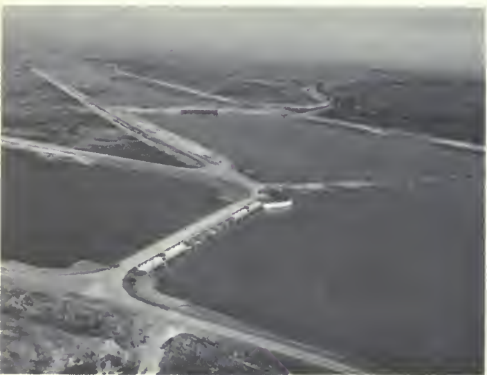
The 14-bay Mariposa Bypass Control structure discharging flow from the Eastside Bypass into the Mariposa Bypass.
