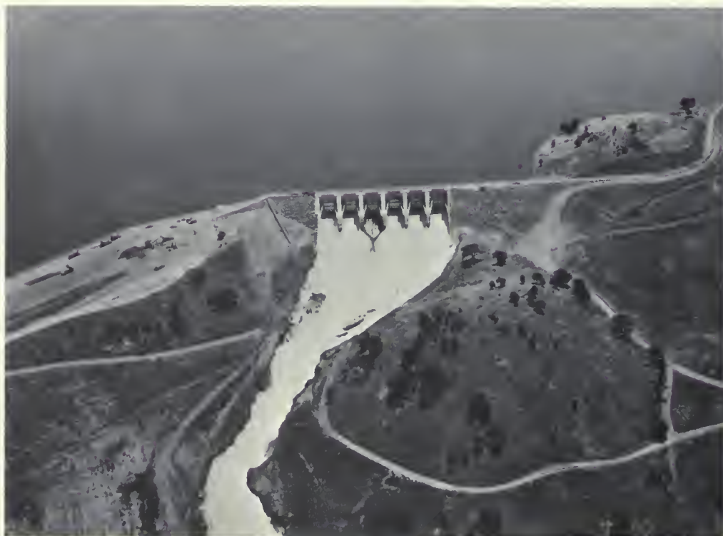
New Exchequer Dam spillway during snowmelt period, June 1966
