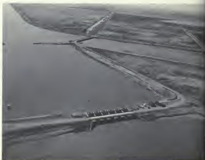
Excess flows being diverted through the six-bay radial-gated Eastside Bypass control structure.
