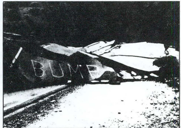
Portions of Hwy 20 shoved nearly 20 ft into air by mile-long mud slide
