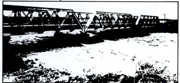
Raging waters of Calleguas Creek batters bridge at Hueneme Rd.
