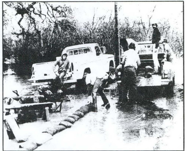
Sandbagging north of Hamilton City
