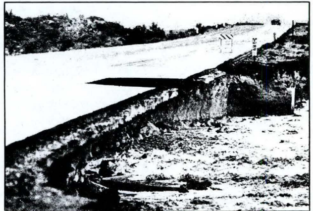
Interstate 8, linking San Diego and Phoenix, is undercut by flood waters just outside Ocotillo.
