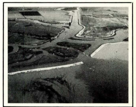
ON THE COVER: McDonald Island Levee Break during flooding in the Sacramento-San Joaquin Delta, August 28, 1982.
