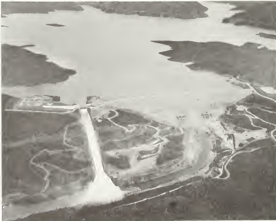
Flood Control Releases at Oroville Dam. DWR Photograph
