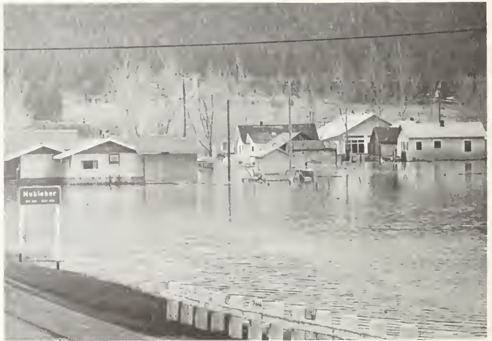
A levee break caused the town of Nubieber to be inundated.
