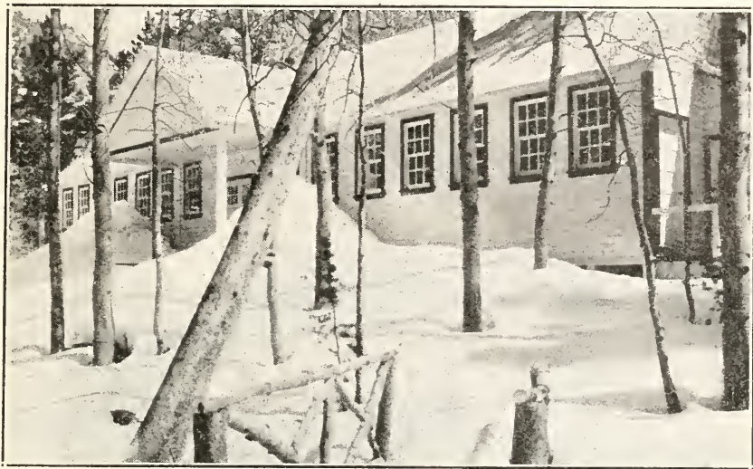
FIG. 16. The new Fern Creek Hatchery, as it appeared in the spring of 1927.
