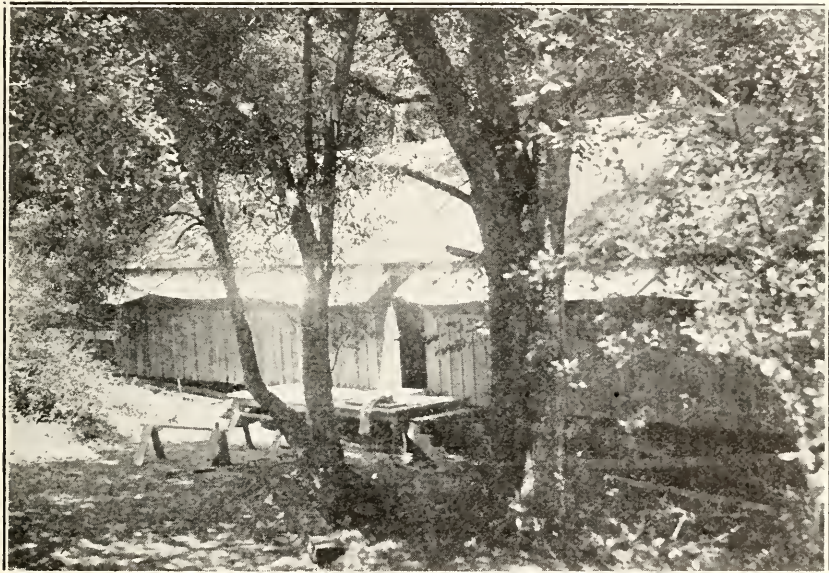
FIG. 13. San Gabriel River Holding Tanks. Better distribution of fish is expected as a result of a number of holding tanks of this type which have been built in various parts of the state.
