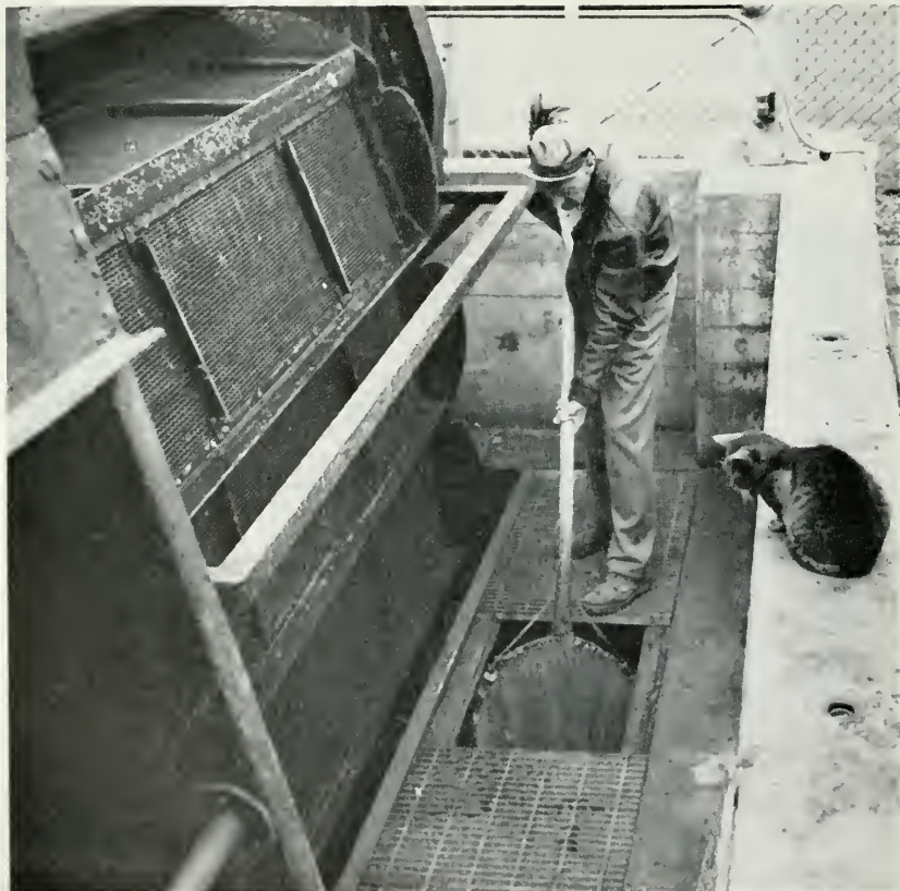
FIGURE 2. The junior author hoisting up the collecting net from the sump in front of the revolving trash screen. Photograph by Toshio Asaeda, November, 1954.
