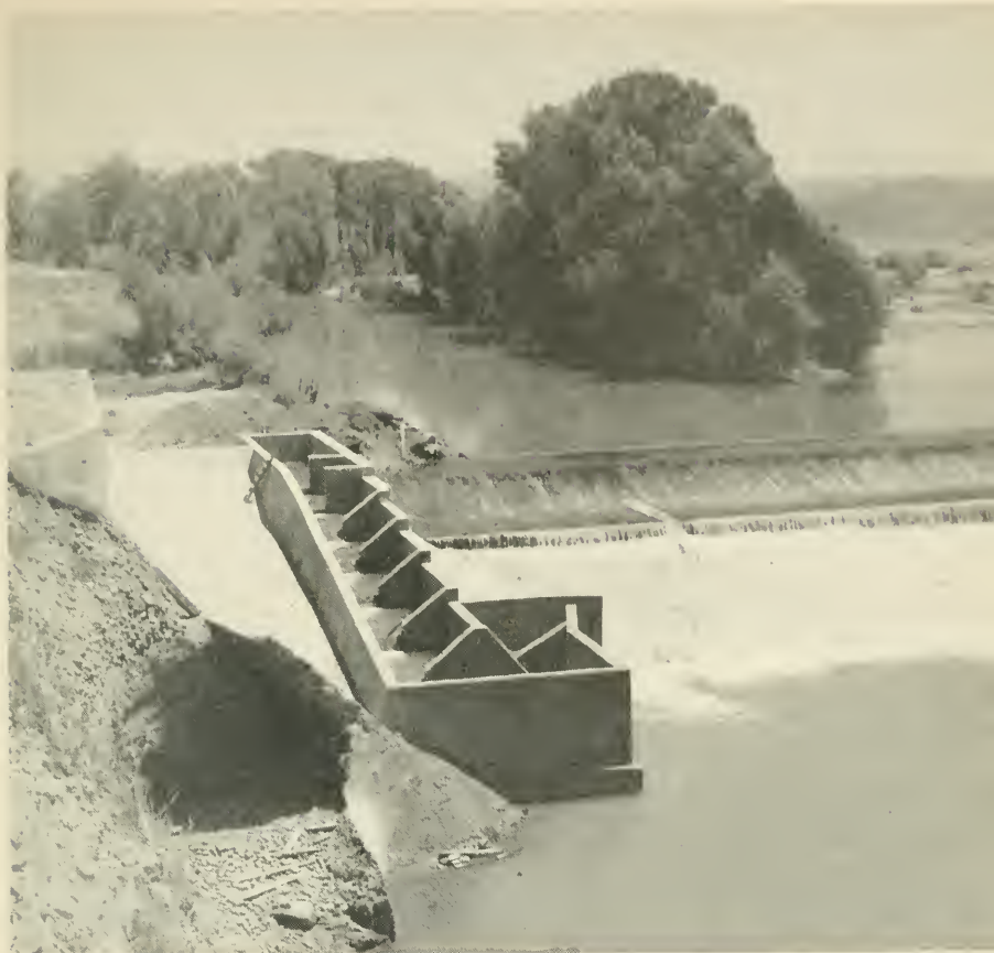
FIGURE 2. The new ladder at the south end of the Daguerre Point dam
