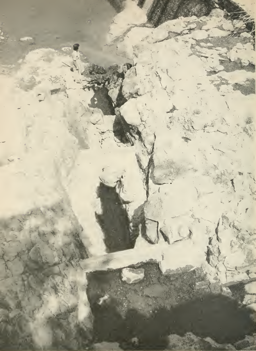
FIGURE 1. Remains of the old ladder at the south end of the Daguerre Point dam, Yuba River. Photograph by D. H. Fry, Jr.
