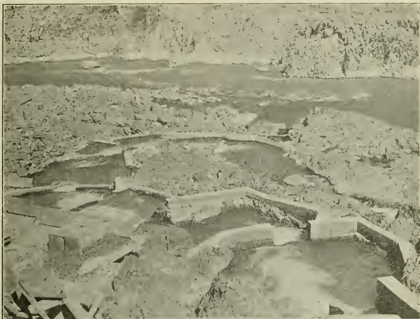
Fig.49. Fish ladder at Snow Mountain dam, Mendocino County. Investigation has shown that fish readily ascend this ladder.
