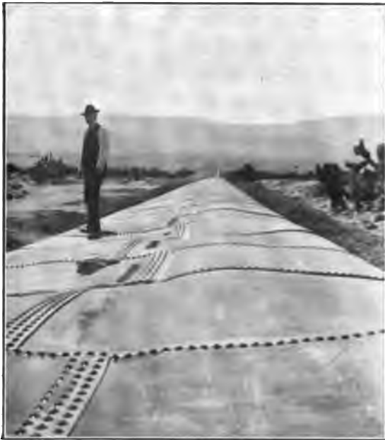
Partly Restored to Form
