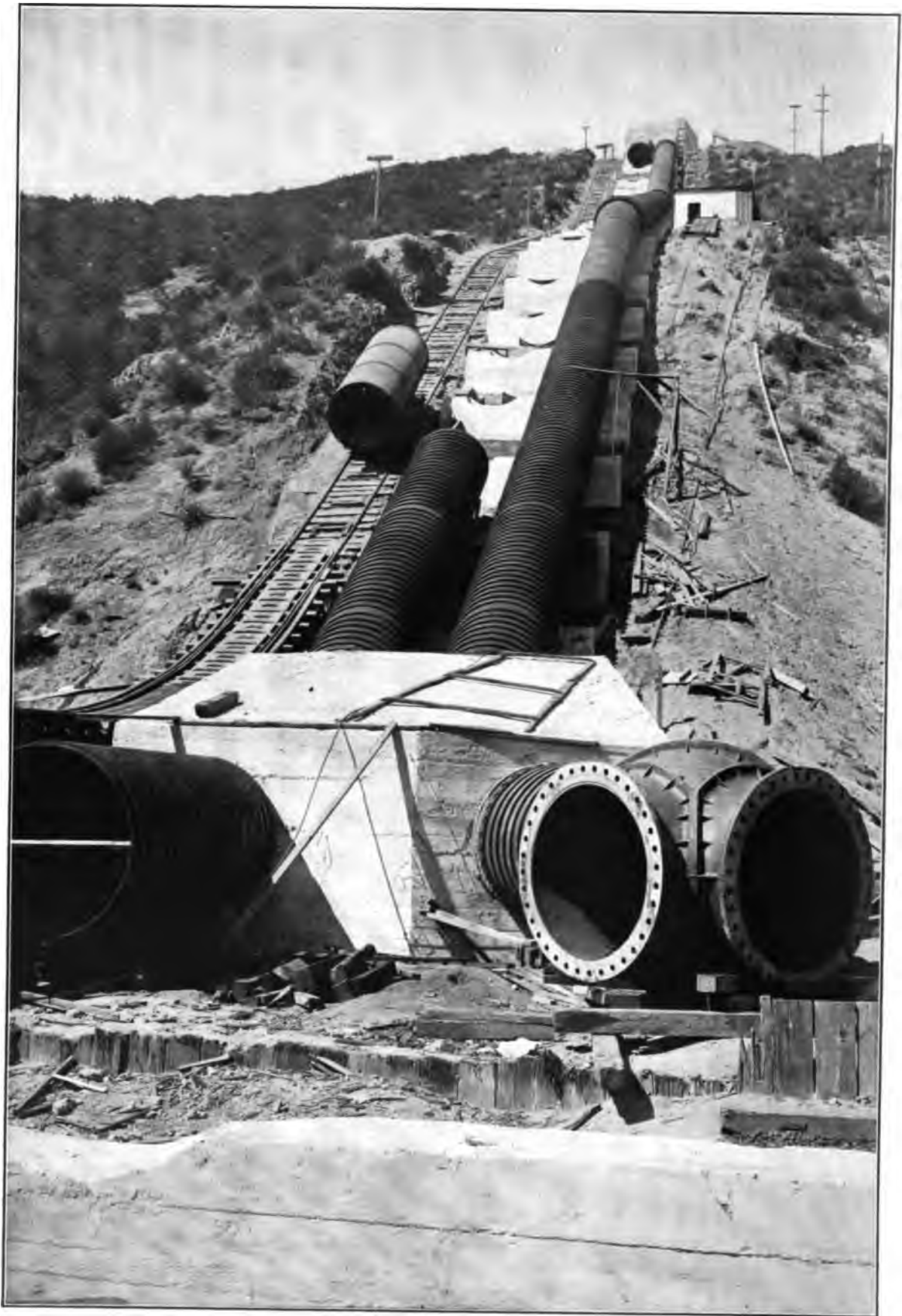
PART OF PENSTOCK OF POWER PLANT NO. 1
