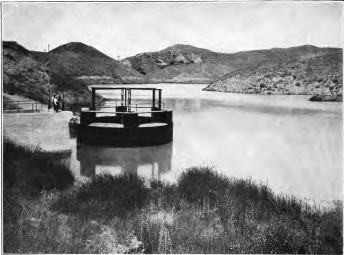
DRY CANYON RESERVOIR, SHOWING FLOATING WEIR
