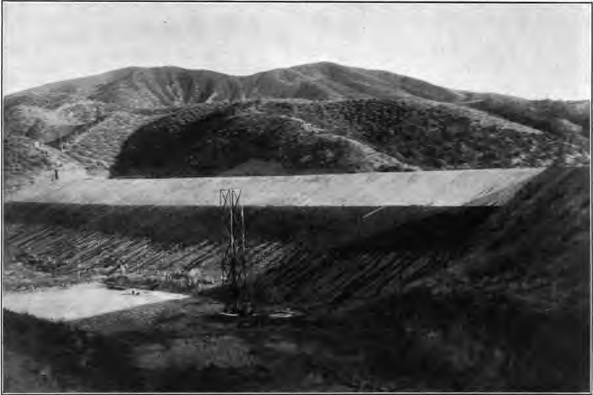
UPSTREAM FACE OF CANYON DAM
