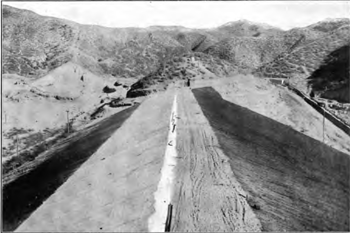
Dry Canyon Dam, Looking East, Showing Finished Structure. The Wasteway of the Reservoir is visible in the Background
