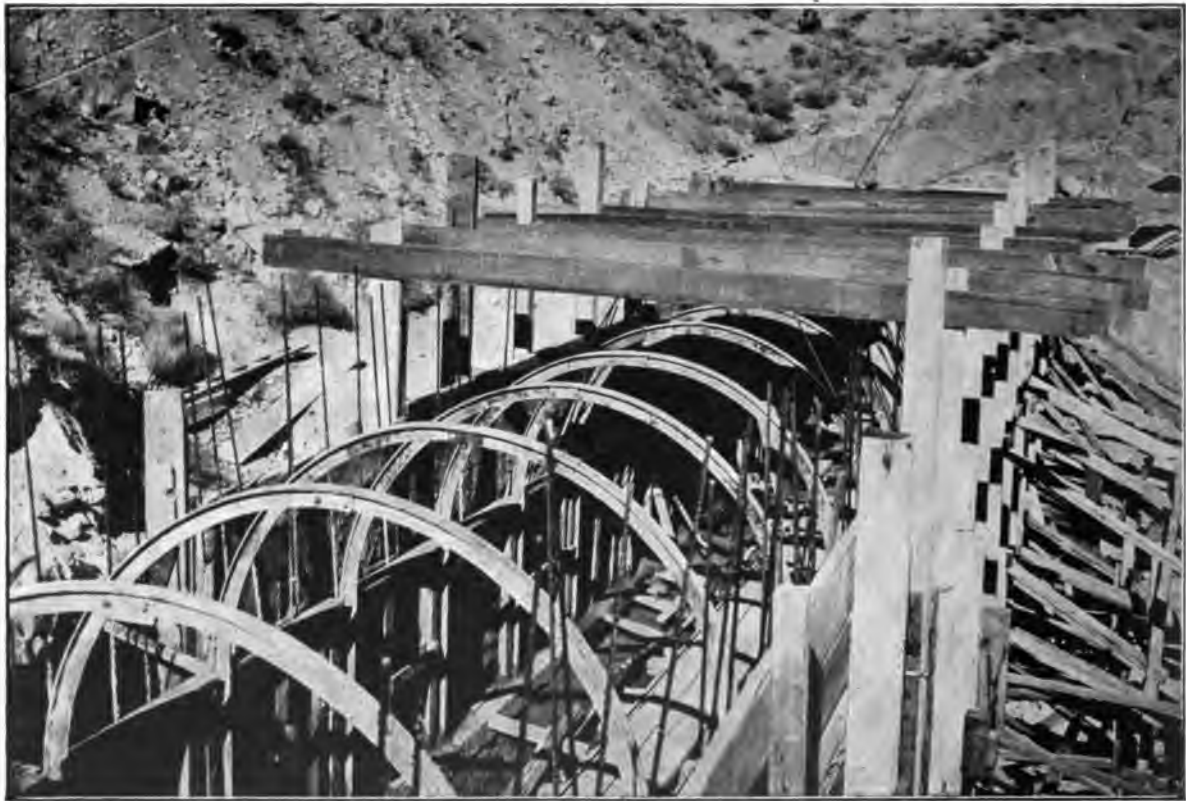
Short Section of Aqueduct Between Tunnels Where Tunnel Forms Were Used
