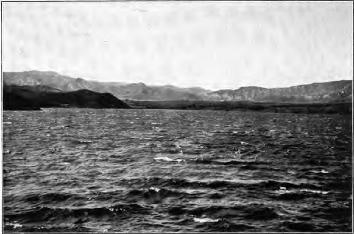
VIEW OF SAN FERNANDO RESERVOIR FROM DAM
