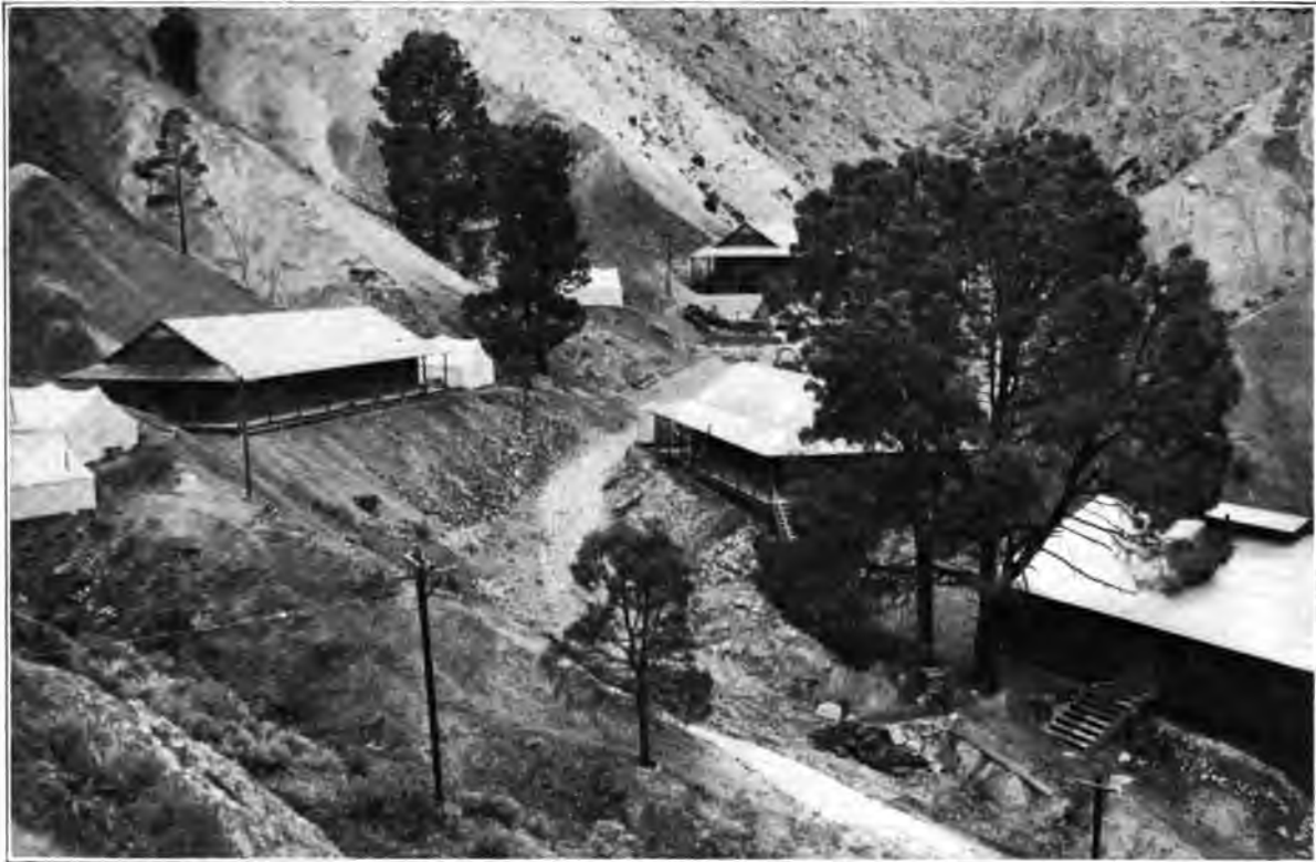
CONSTRUCTION CAMP IN WATER CANYON, JAWBONE DIVISION
