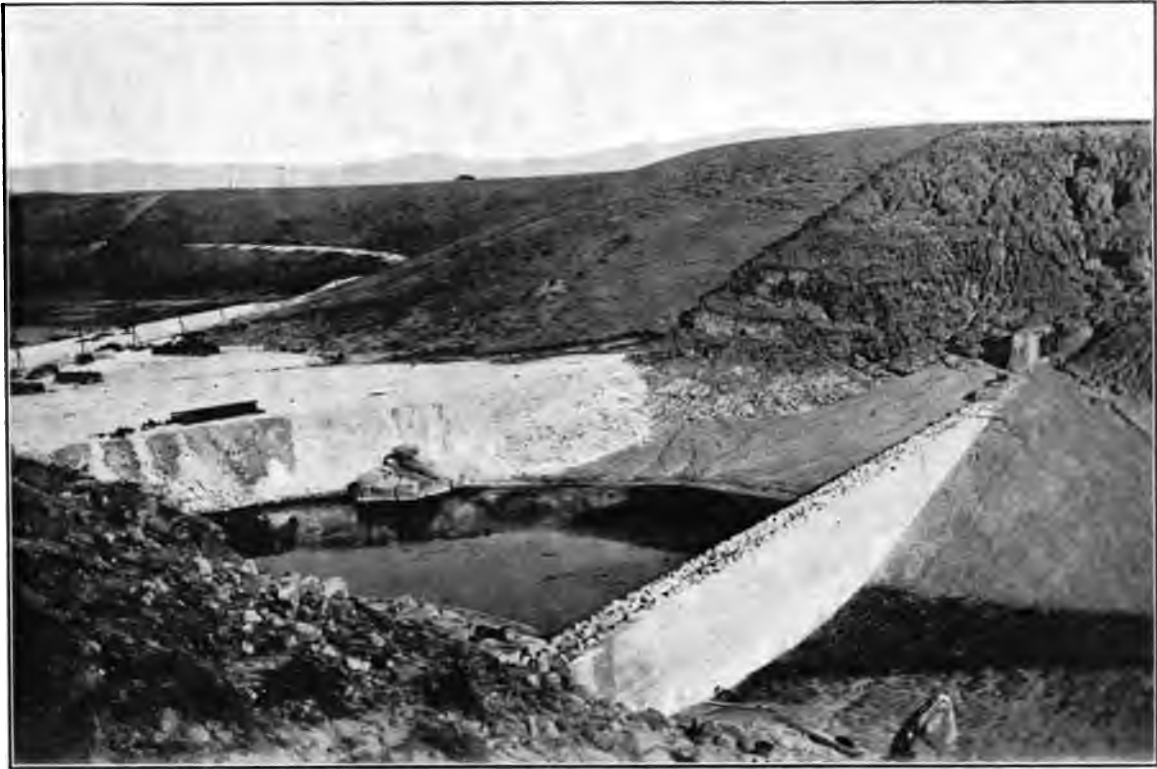
CORE WALL OF FAIRMONT DAM (Unfinished)
