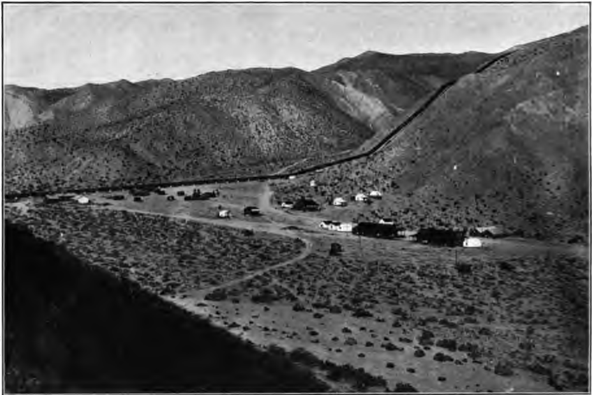
NORTH END OF PINE CANYON SIPHON
