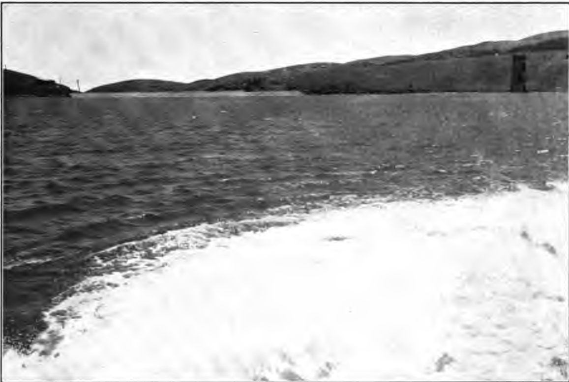
FAIRMONT RESERVOIR, LOOKING SOUTH FROM INTAKE
