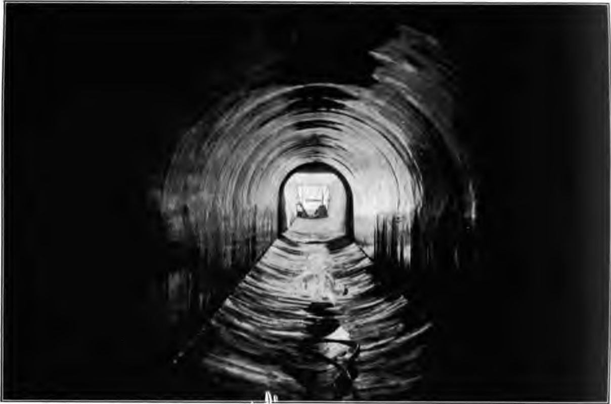
A Lined Tunnel in the Saugus Division
