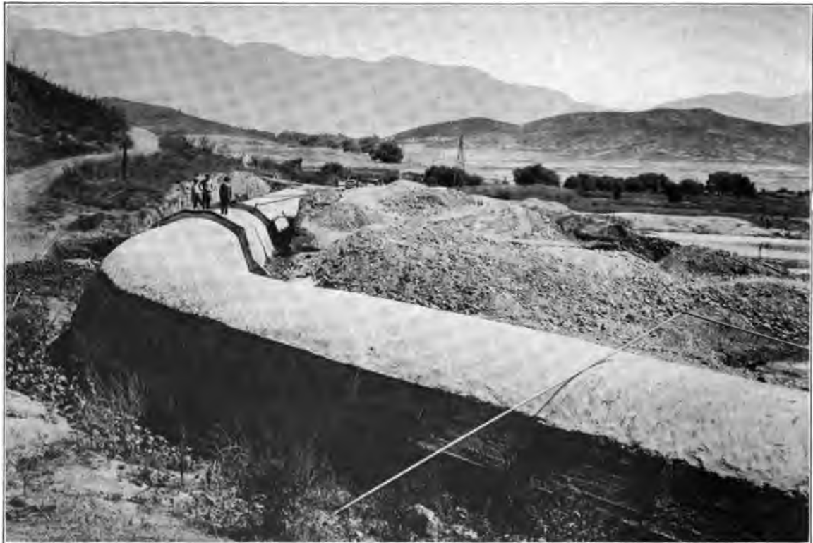
OUTLET TUNNEL OF LOWER SAN FERNANDO RESERVOIR
