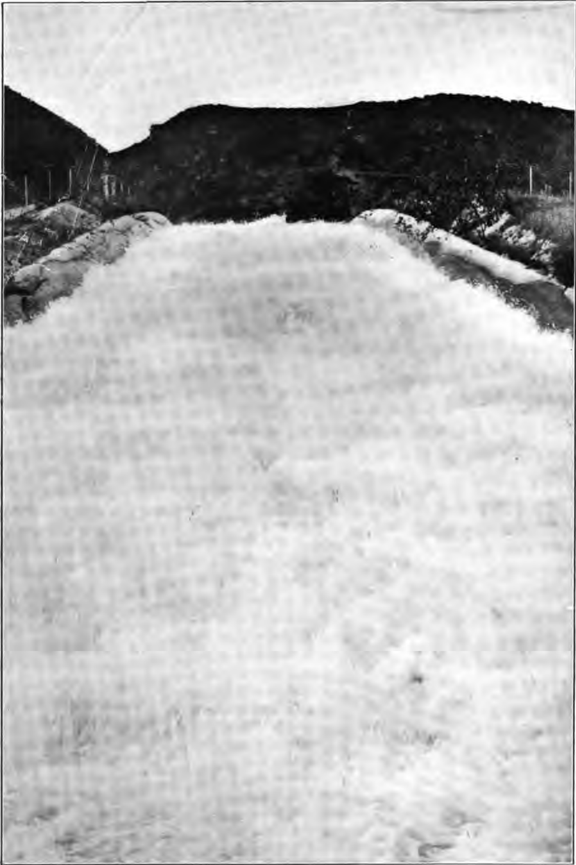
Close View. Head of Cascade at Outlet of Los Angeles Aqueduct.
