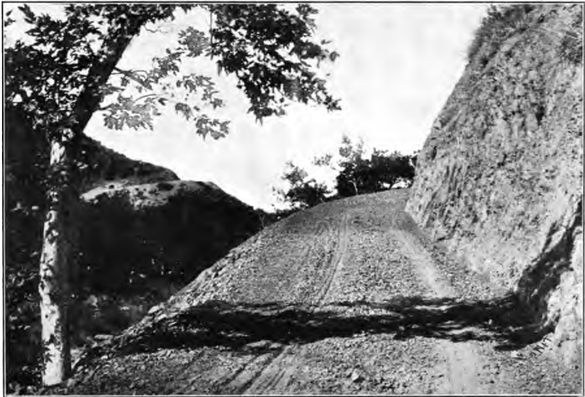
A CONSTRUCTION ROAD IN SAN FRANCISQUITO CANYON
