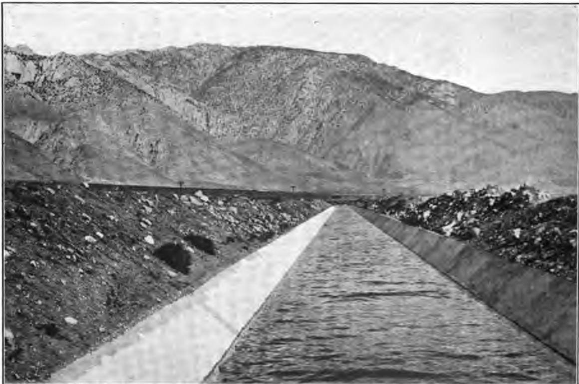
OPEN LINED CANAL IN OLANCHA DIVISION
