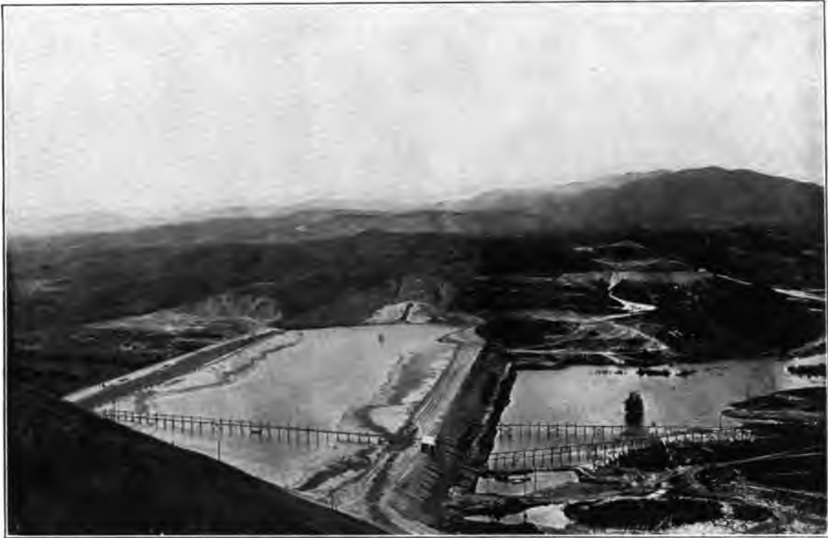
Construction of Lower San Fernando Dam, July, 1913
