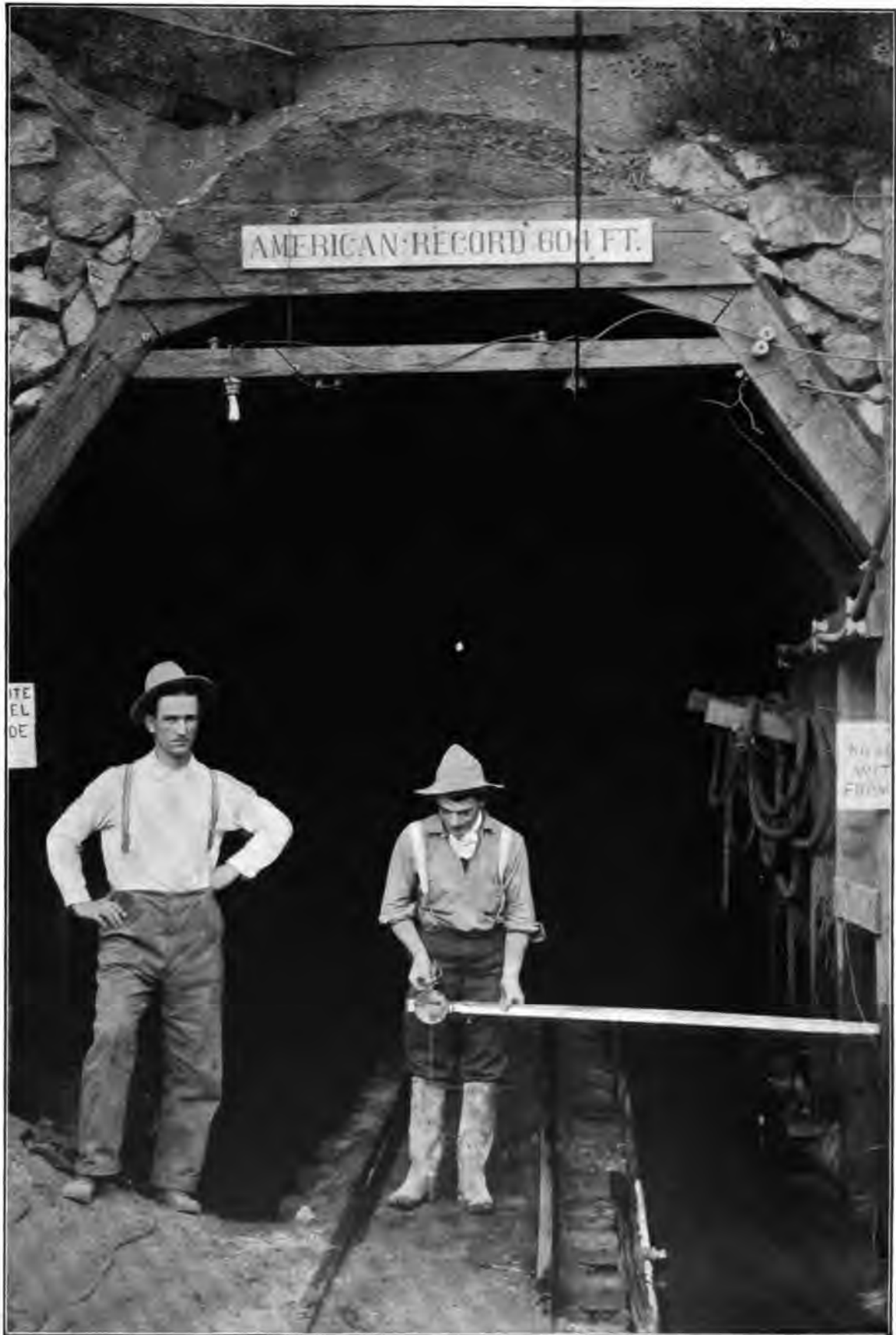
PORTAL OF ELIZABETH TUNNEL, WHERE AMERICAN HARD-ROCK RECORD WAS MADE
