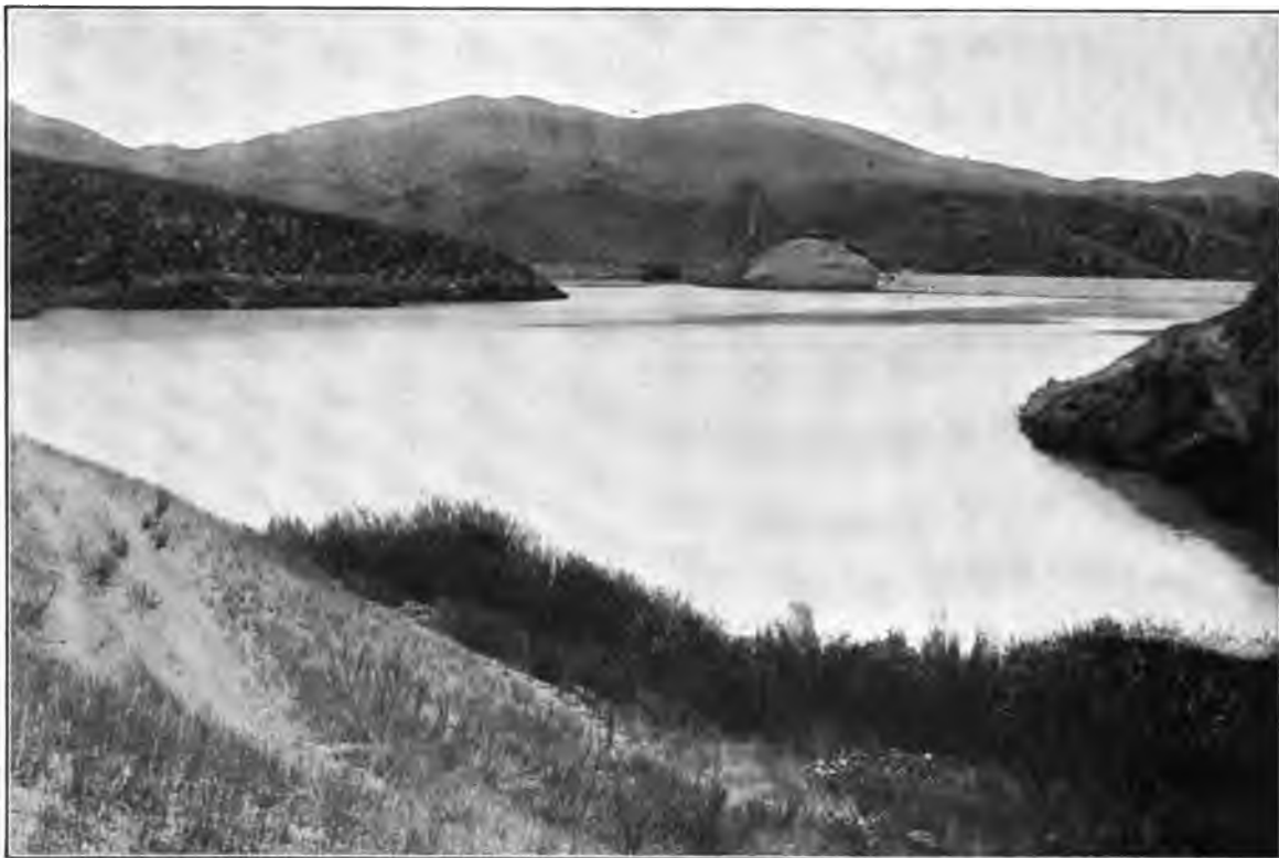
DRY CANYON RESERVOIR PARTLY FILLED
