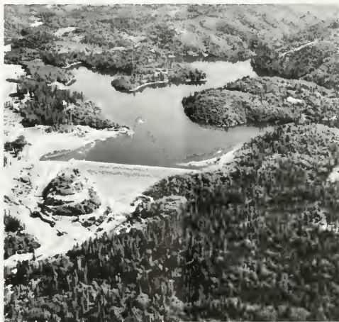
Rollins Dam on Bear River
