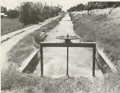
Natomas Ditch in Sacramento County
