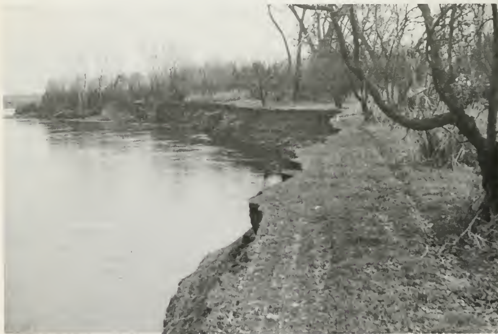
Bank erosion—a continuing problem
