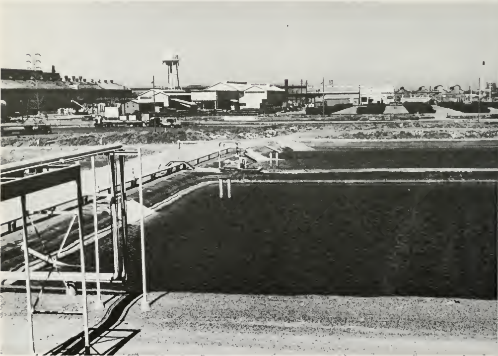
Water quality protection through evaporation of toxic waste Dow Chemical Co. photo
