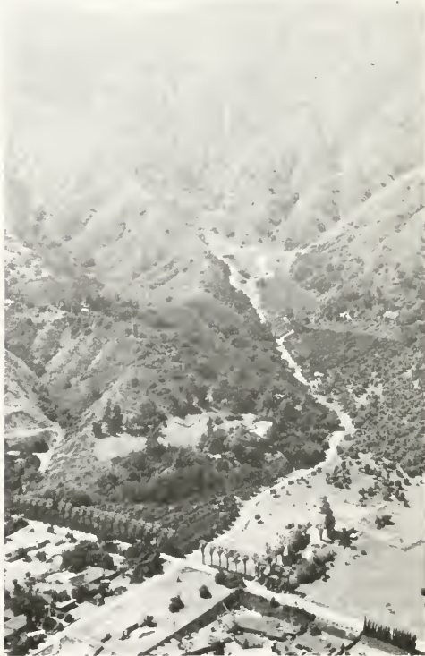
Urban development below debris control structure
