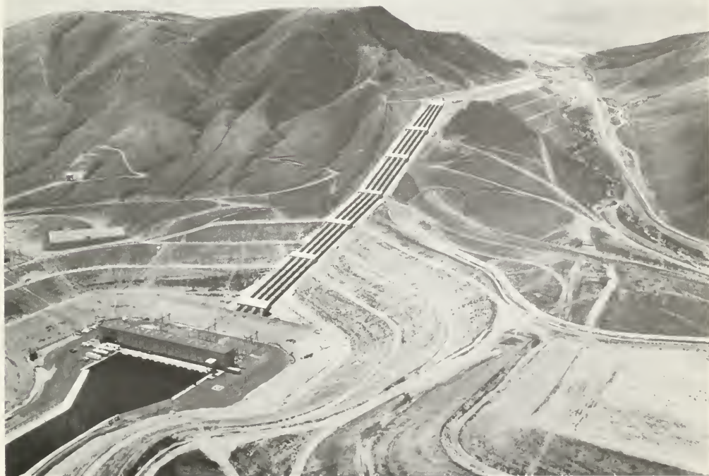
Wind Gap Pumping Plant—California State Water Project
