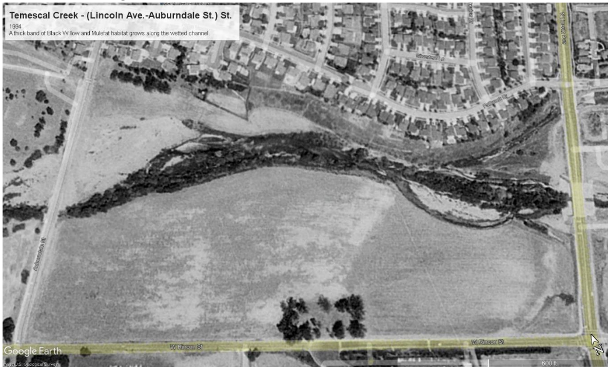
Figure 3. 1994 Temescal Creek – Lincoln Ave. to Auburndale St.
