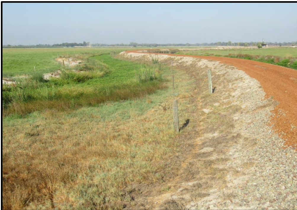
East part of potential GDE #3212, looking west from on top of an access road; 09/03/21. This portion of potential GDE is comprised of the edge of a field, a private agricultural drain, MID's maintenance road, and the south edge of MID's drainage canal.
