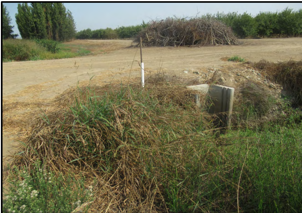
Potential GDE # 7705 (Riley Slough), looking northeast; 09/15/21. There are control gates and valves along the length of this agricultural drain, allowing water levels to be adjusted for irrigation, drainage, and/or conservation purposes.
