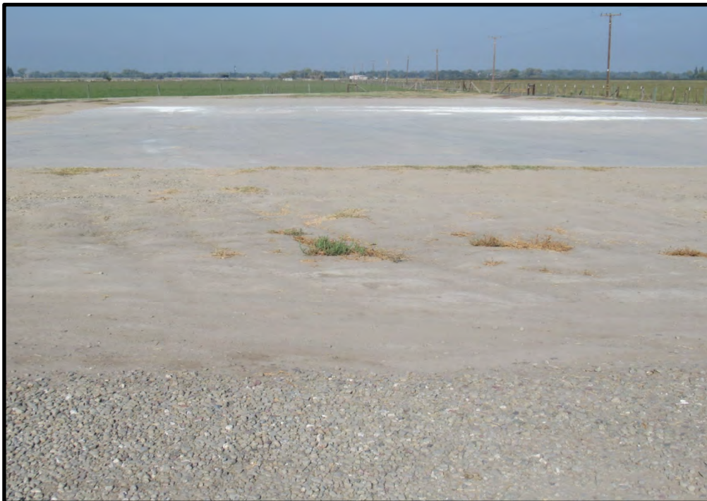
Potential GDE #7785, looking west from the east end of the concrete pad; 09/03/21. This potential GDE comprises the concrete pad, adjacent gravel areas, and a sliver of the MID lateral.
