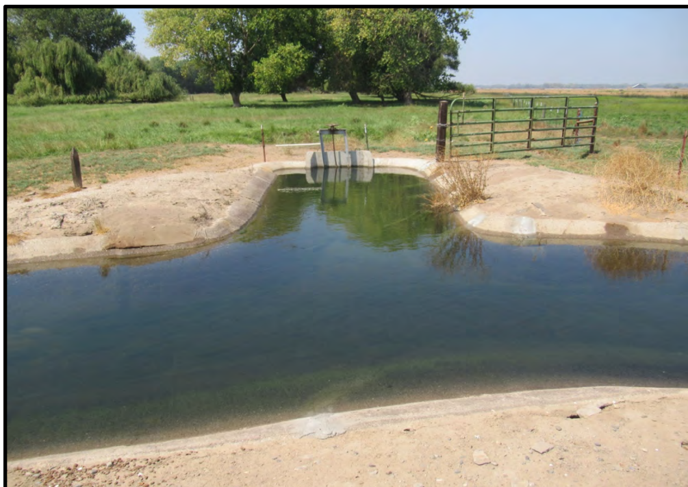
Gate valve along the MID lateral that can be opened to provide water to a cluster of constructed habitats to the west (i.e., potential GDEs # 7755, 7757, 7758, 7759, 7761, 7767, 7768, 7769, and 7771), looking northwest; 09/03/21.
