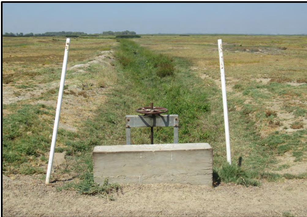
Water being conveyed from the MID lateral and/or groundwater wells via a pipeline in to potential GDE #7748, looking northwest; 09/03/21.
