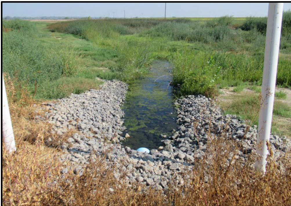
Potential GDE #7763, looking northeast; 09/03/21. This shallow basin is only a few feet deep and can be filled by opening a valve from a private lateral. This area has been graded to provide upland and wetland habitats and is managed for conservation.
