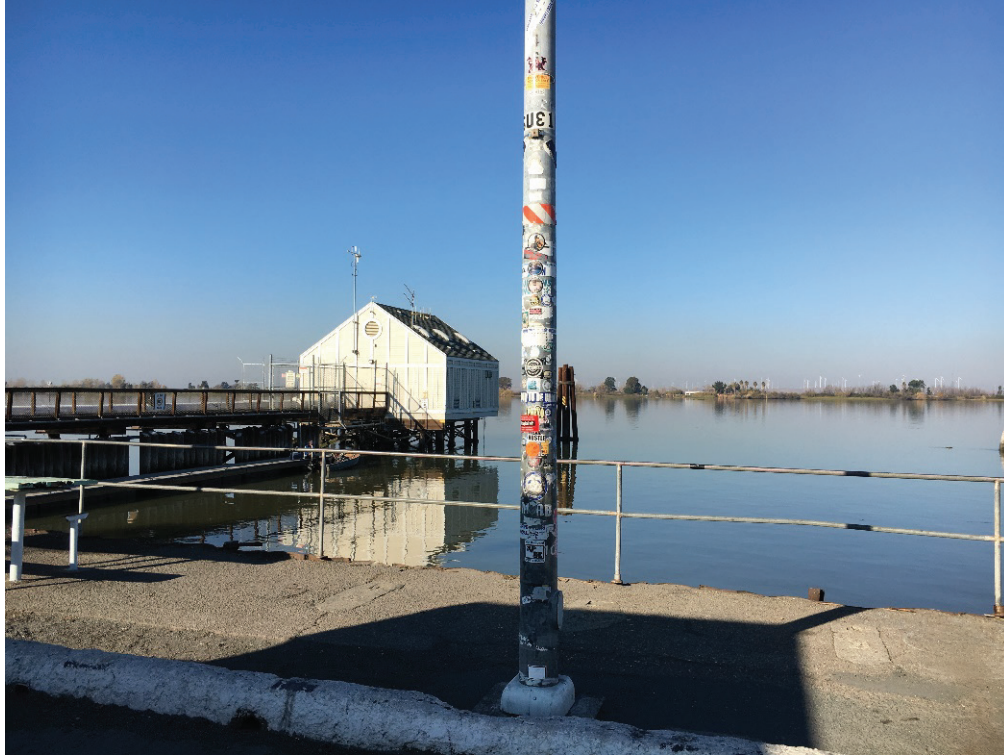
View 1: Existing river intake pump station. View facing north.
