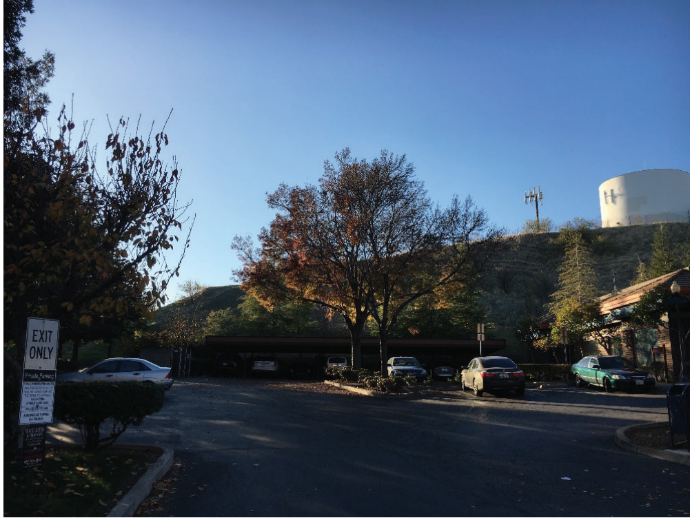
View 3: View toward Antioch Water Treatment Plant (WTP) from View Drive. View facing northeast.
