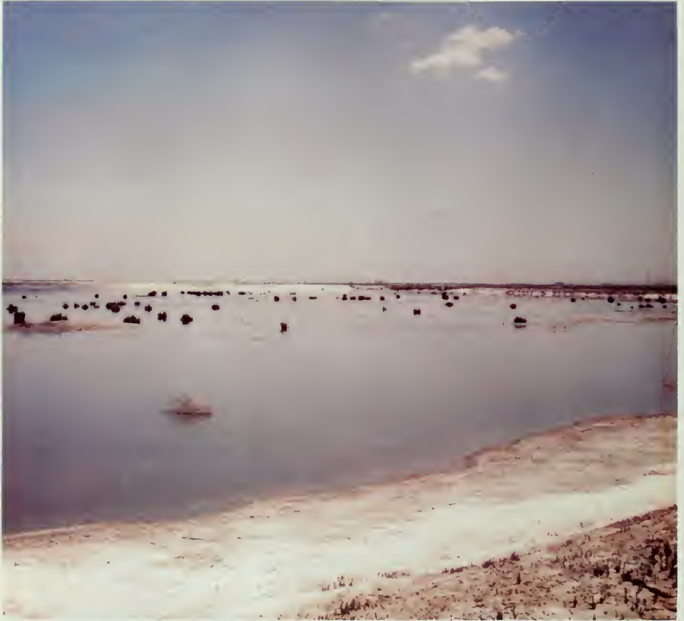
In the absence of a drainage export facility, evaporation ponds are used as salt sinks to dispose of drainage water too salty for reuse.
