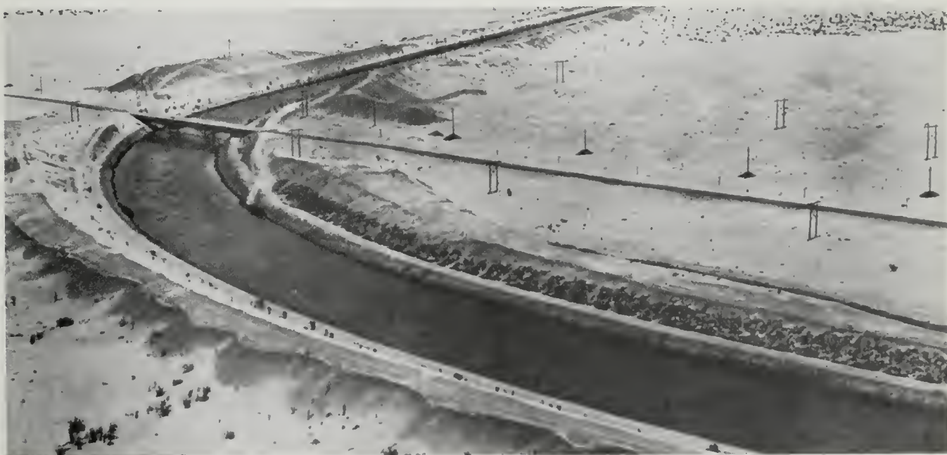
After leaving the Colorado River, the All-American Canal crosses an expanse of desert to reach the Imperial Valley.
