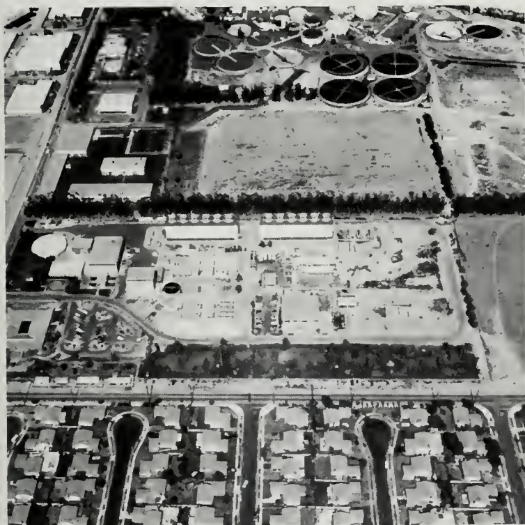
Water Factory 21 in Orange County. Operation of this plant, together with the primary and secondary treatment of municipal waste water at the plant appearing at top, involve most of the treatment processes in use today. Treated water produced by advanced treatment and desalted water are blended with water from deep wells and then injected underground to form a barrier to sea water intruding into the ground water in the region.
