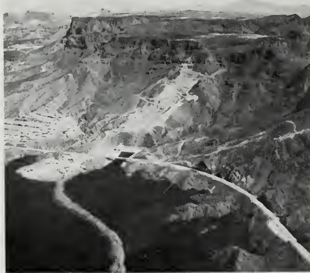
Havasu Pumping Plant at Lake Havasu on the Colorado River, a facility of the Central Arizona Project. Full use is expected by 1990, at which time California can no longer depend on receiving more than 4.4 million acre-feet per year.
