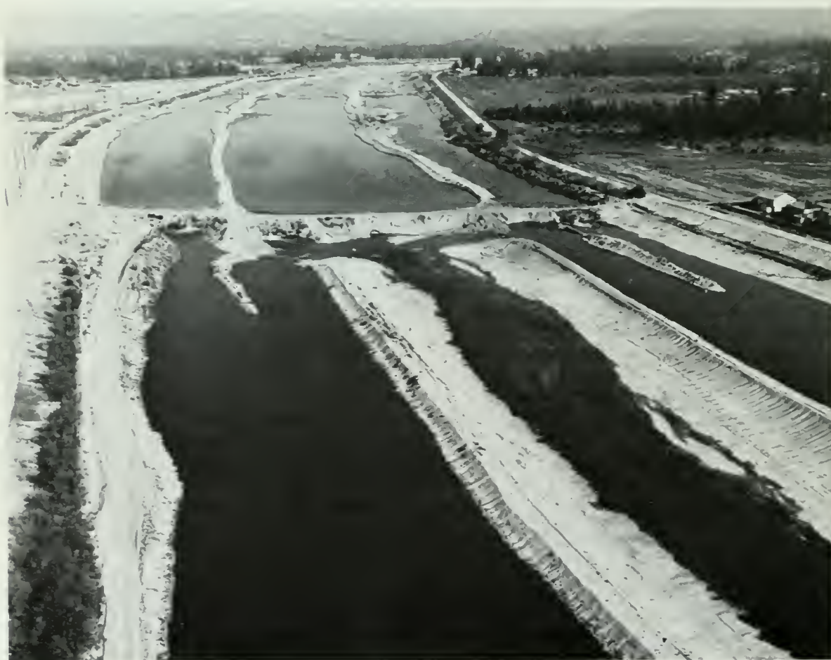
Santa Ana River spreading grounds, a typical ground water recharge operation. Local runoff regulated by Prado Reservoir is replenishing the Orange County ground water basin. The facility could be used in summer to spread surplus SWP water, when it is available.
