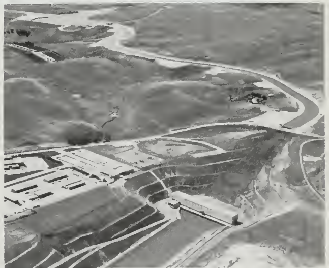
Harvey O. Banks Delta Pumping Plant near Tracy, an SWP facility, lifts water from the Delta 244 feet into the California Aqueduct. The Delta Operations and Maintenance Center is situated at left, and Bethany Dam and Reservoir appear at top. Addition of the final four pumps to bring the plant to design capacity of 10,300 cubic feet per second will improve operational flexibility and provide additional supplies for the SWP.
