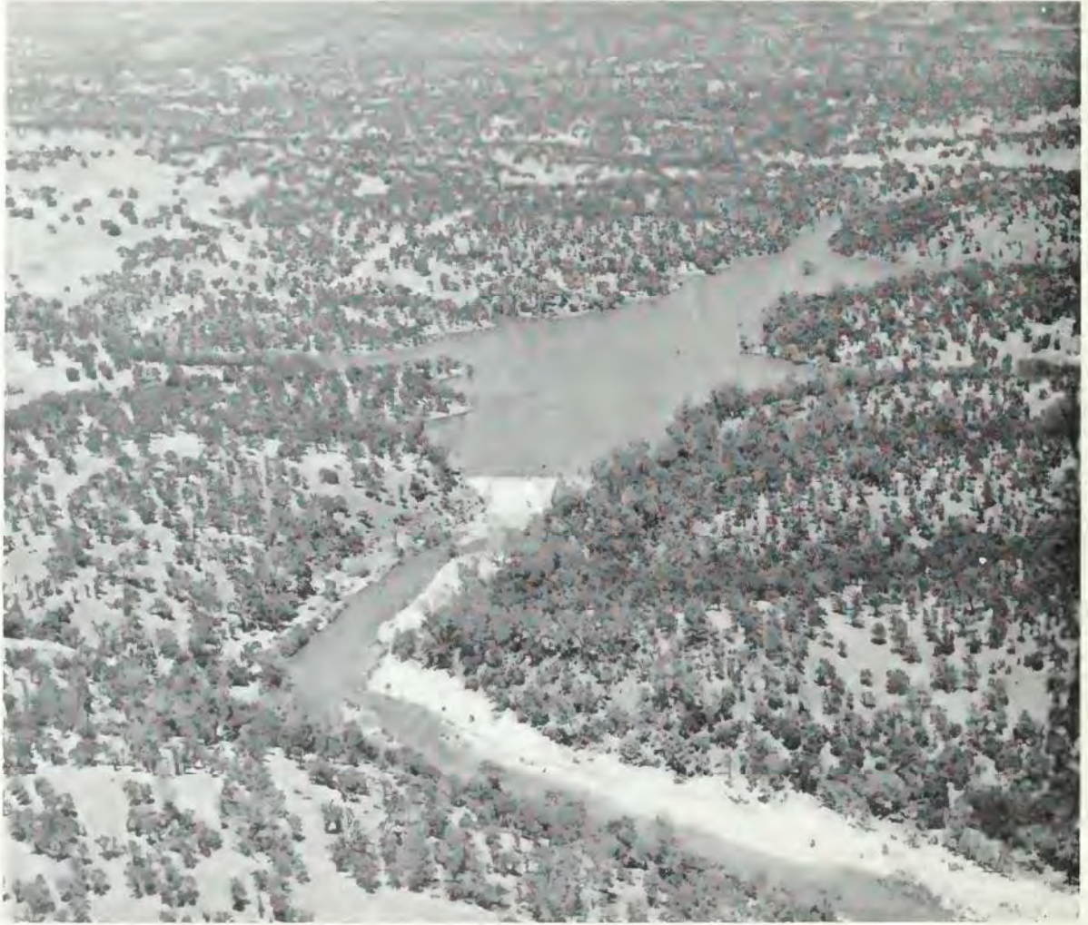
Existing Camp Far West Dam and Reservoir
