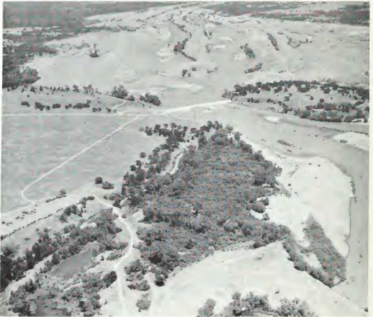
Daguerre Point Weir on Yuba River
