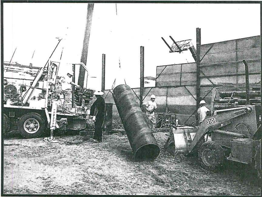
Installing 36-inch conductor pipe
