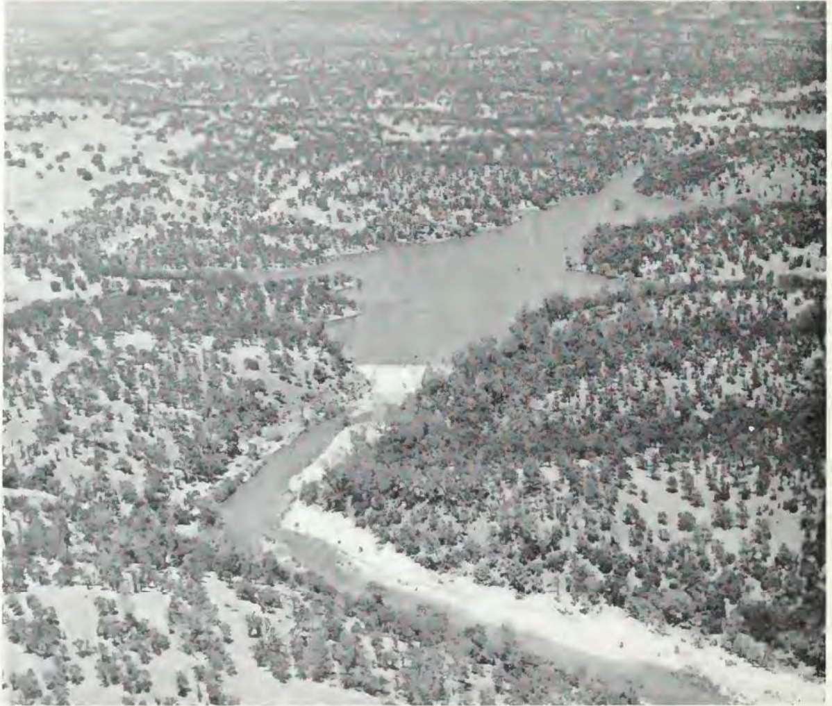
Existing Camp Far West Dam and Reservoir
