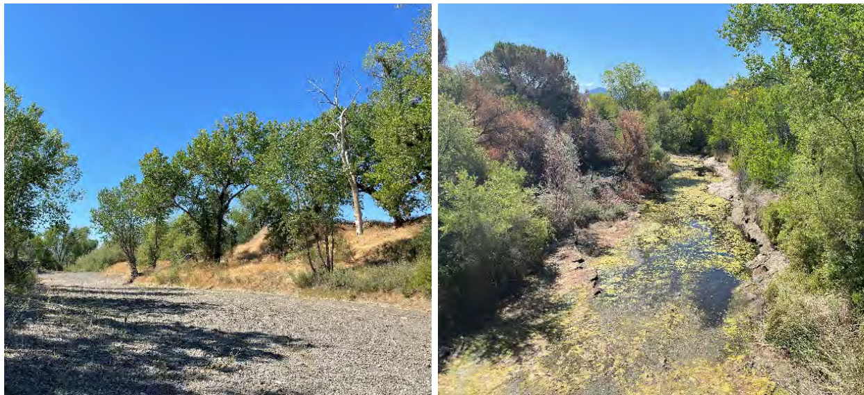
Figure 2-43. Kelsey Creek Channel Downstream (left) and Upstream (right) from the Main Street Bridge
