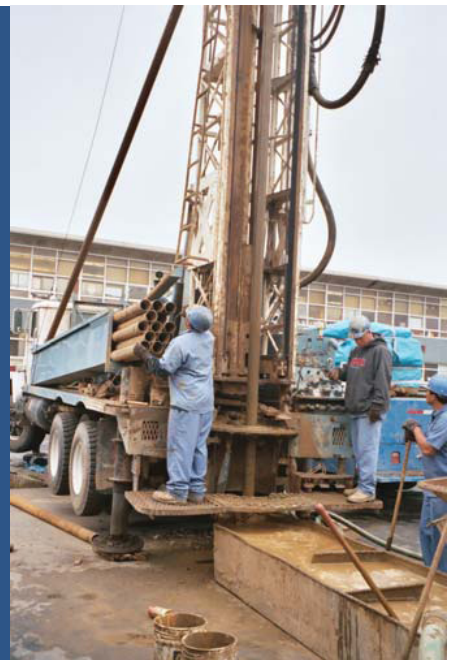
Drilling operation for nested monitoring well
