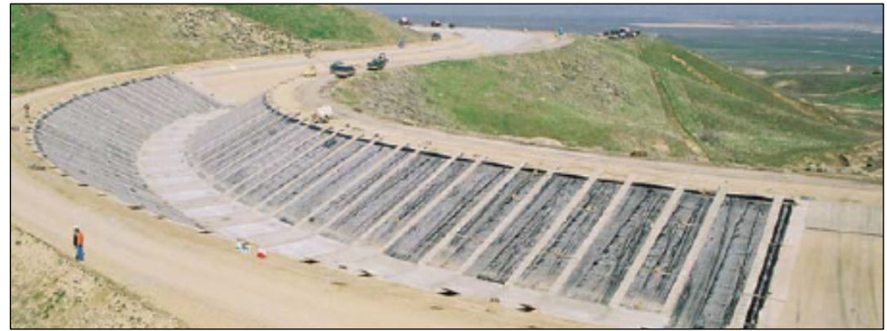
Lining of California Aqueduct Canal in Southern California in 1999
