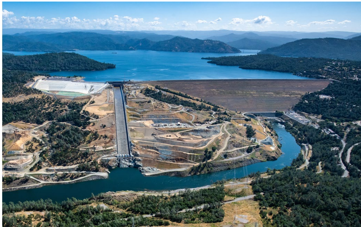
Figure 2. Facilities of Oroville Dam, Including Main Dam Embankment, Flood Control Outlet Spillway, and Roller-Compacted Concrete Apron below Emergency Spillway Crest (DWR 2019)
