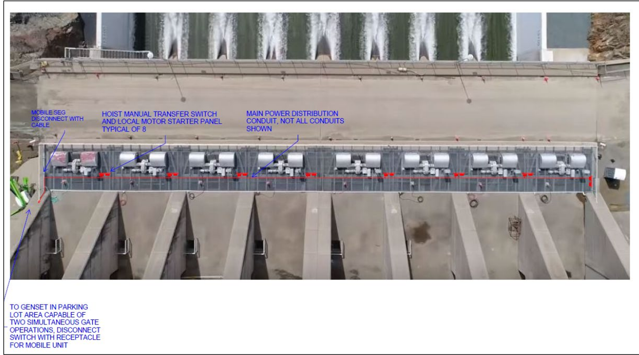
Figure 26. Recommended Interim Implementation Project Measure—Install Backup Power and Remote Starters for FCO Radial Gates (Measure T3-BH.2)
