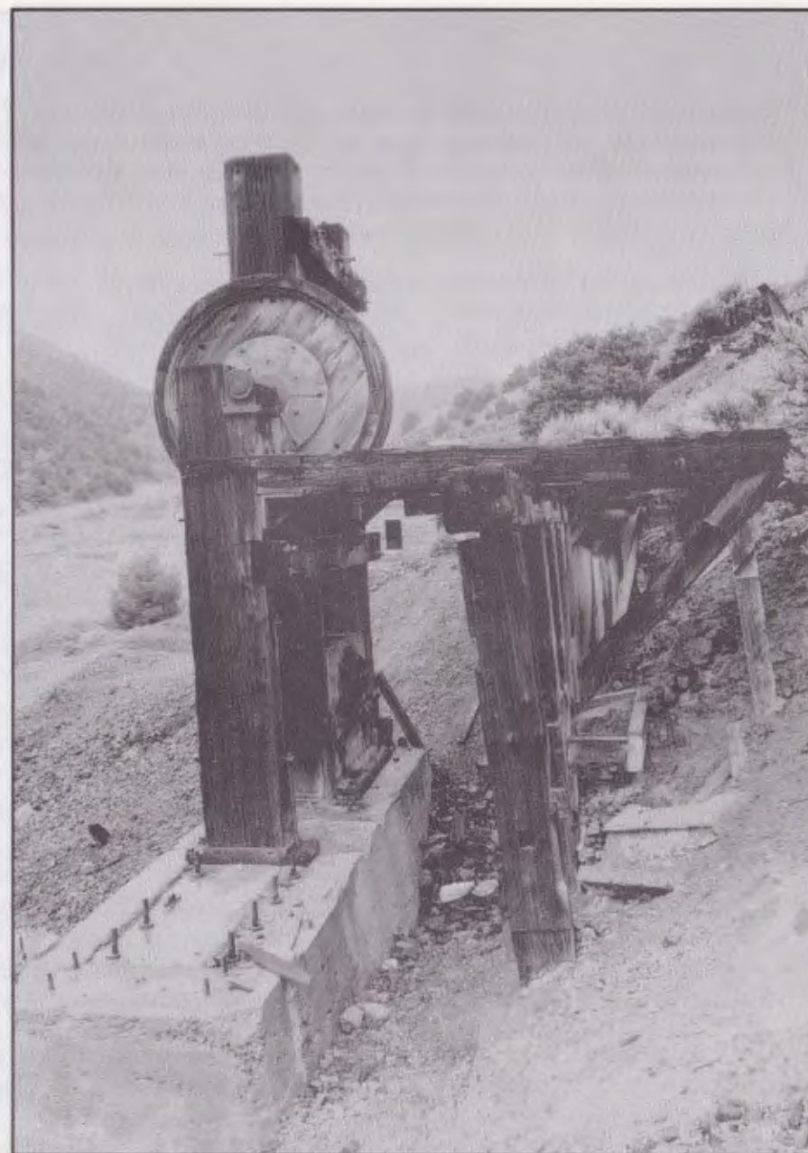
The remains of a stamp mill at Pine Grove. The large wooden wheel was turned by a belt connected to a shaft powered by steam or water. The rotation of the wheel would lift the stamps to crush the ore. The stamps have been removed from this mill, but their crankshaft remains.
