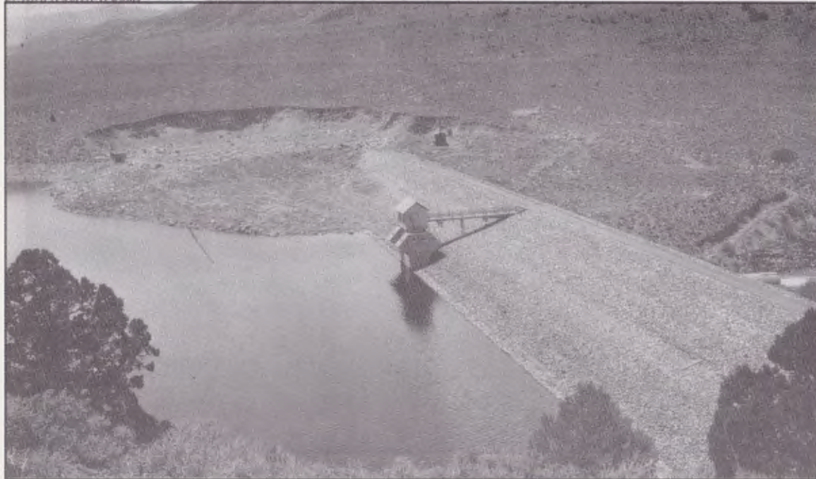
A 1931 bird's eye view of Bridgeport Dam showing both its spillways. The primary spillway, the structure seen on the embankment, is an uncommon type of siphon spillway. The borrow pit used during dam construction (at upper left) also serves as the auxiliary spillway.
