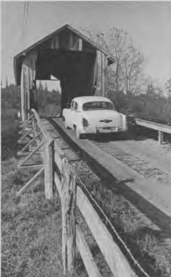
ONE OF THE FEW covered bridges still left in California, this structure crosses the Elk River at Fields Landing. Considerable lumbering activity took place in this area during the late Nineteenth Century.
