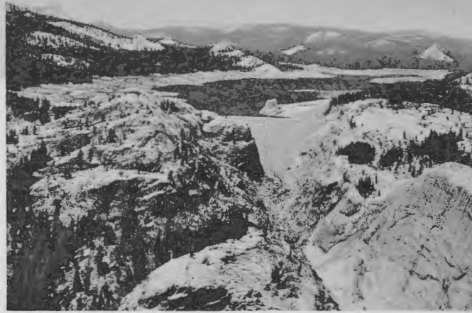
COURTRIGHT RESERVOIR 8,184 feet above sea level, stores 123,300 acre feet of water as part of Kings River hydraulic project. Rising 300 feet above the stream bed, the dam contains 1,564,000 cubic yards of rock. Peaks more than 13,000 feet high in the background.
