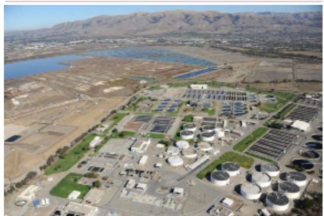
Figure 3.3 Coastal wastewater treatment facilities, many of which are located at sea level, are increasingly at risk of being compromised by flooding due to sea-level rise. (Photo: San Jose-Santa Clara Regional Wastewater Facility; Land Use Interpretation Center ; licensed under Creative Commons license 3.0)
