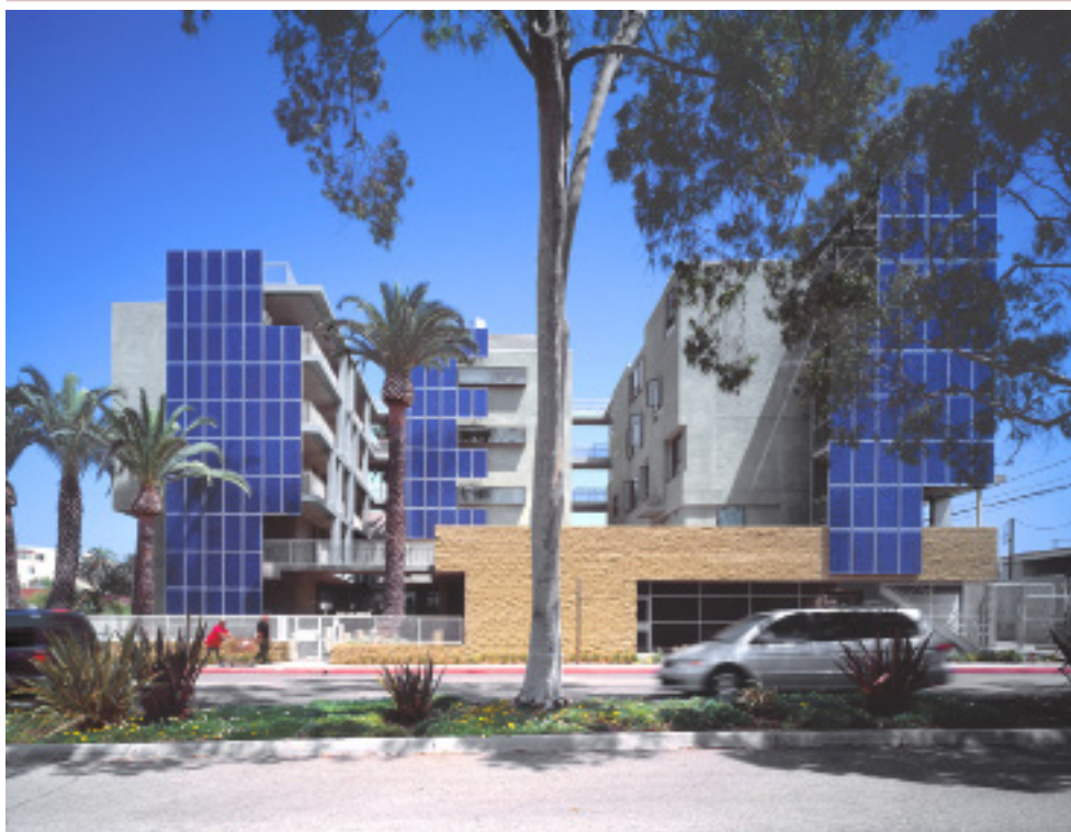
Figure 7.8: Integrated infrastructure development can create many synergies and co-benefits. This multi-family housing unit, known as Colorado Court, in Santa Monica was the first LEED “Gold” certified multi-family building in the U.S. It combines many sustainability features and provides affordable housing to lower-income residents. (Photo: Calder Oliver, Wikimedia Commons , licensed under Creative Commons license 2.0)
