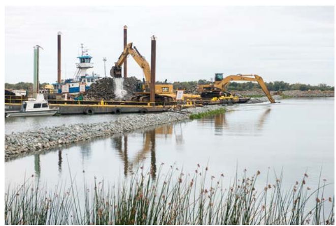
Figure 10.1: A wide variety of barriers make the use of forward-looking climate and other science challenging in infrastructure design. (Photo: Dismantling of a drought barrier along the West False River which served to block salt water from pushing into the central Sacramento-San Joaquin Delta from San Francisco Bay; Florence Low, DWR, used with permission).
