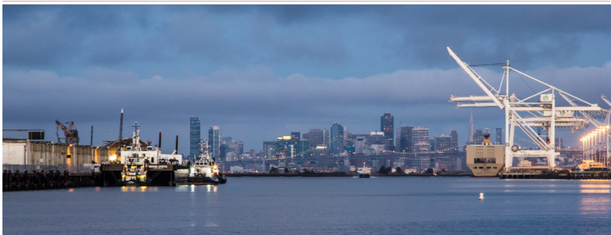
Figure 3.13 Ports, airports and telecommunications infrastructure – while not State-owned – are critically important to the state’s functioning and economy. Many of these infrastructure systems are increasingly at risk from flooding, sea-level rise, wildfires and other extreme events. (Photo: San Francisco skyline and Port of Oakland, Tony Webster, flickr , licensed under Creative Commons license 2.0)
