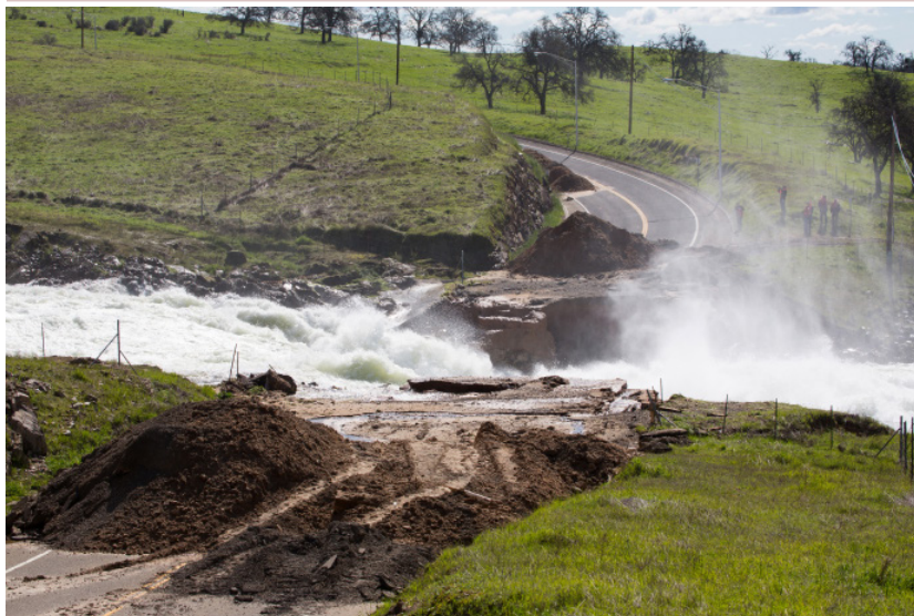
Figure 9.6 In a crisis, expedited permitting is crucial, but rebuilding with climate change in mind must become part and parcel of permitting and waiver guidance. (Photo: Bonds Flat Road near the Don Pedro Dam spillway, February 23, 2017; Dale Kolke, DWR, used with permission)
