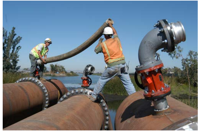
Figure 7.1 Generally, standards are developed at the international and national levels through standard-setting organizations and states and local jurisdictions adopt them. Sometimes, states and local governments develop more stringent codes and standards that go above and beyond minimum standards. (Photo: Pipe installation at Jones Tract levee break in 2004; DWR, used with permission)
