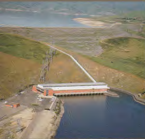
Gianelli Pumping-Generating Plant
