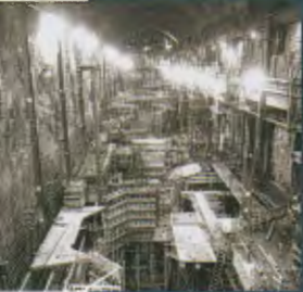
Hyatt Power Plant
