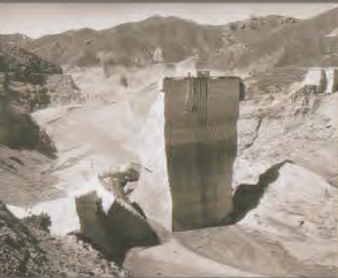
1928 failure of St. Francis Dam.
