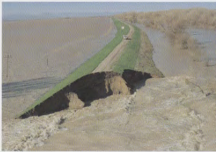
A 300-foot wide levee break at the Jones Tract required around 200,000 to 215,000 tons of rock to fill. The breach allowed about 160,000 acre-feet of water to cover the 12,000-acre island to an average depth of about 12 feet.
