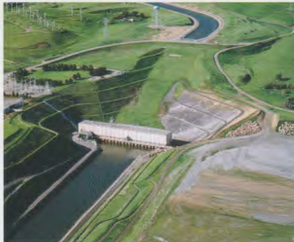
Banks Pumping Plant
