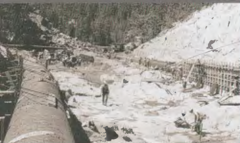
Antelope Facility construction
