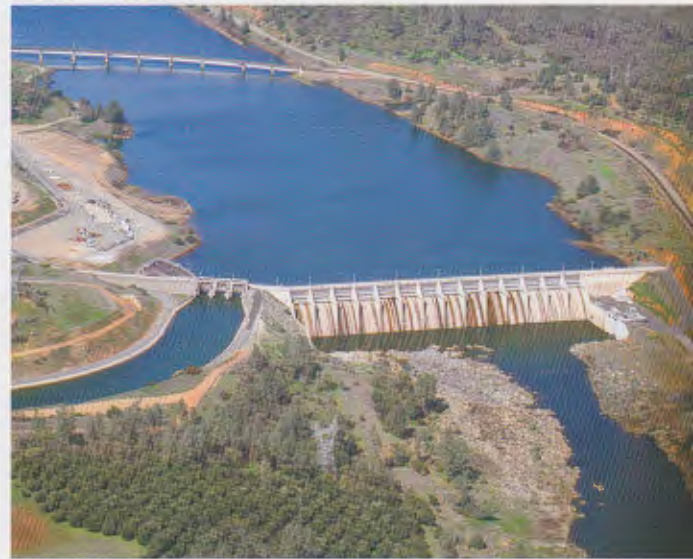
Thermalito Diversion Dam and Powerplant
