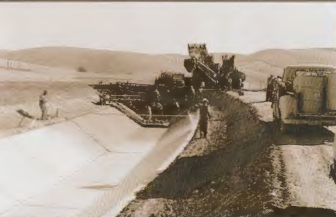
South Bay Aqueduct Construction
