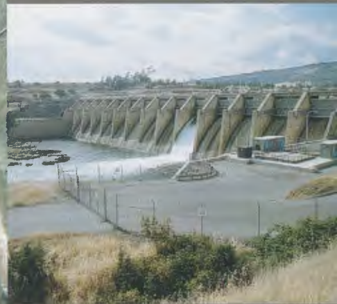
Thermalito Diversion Dam
