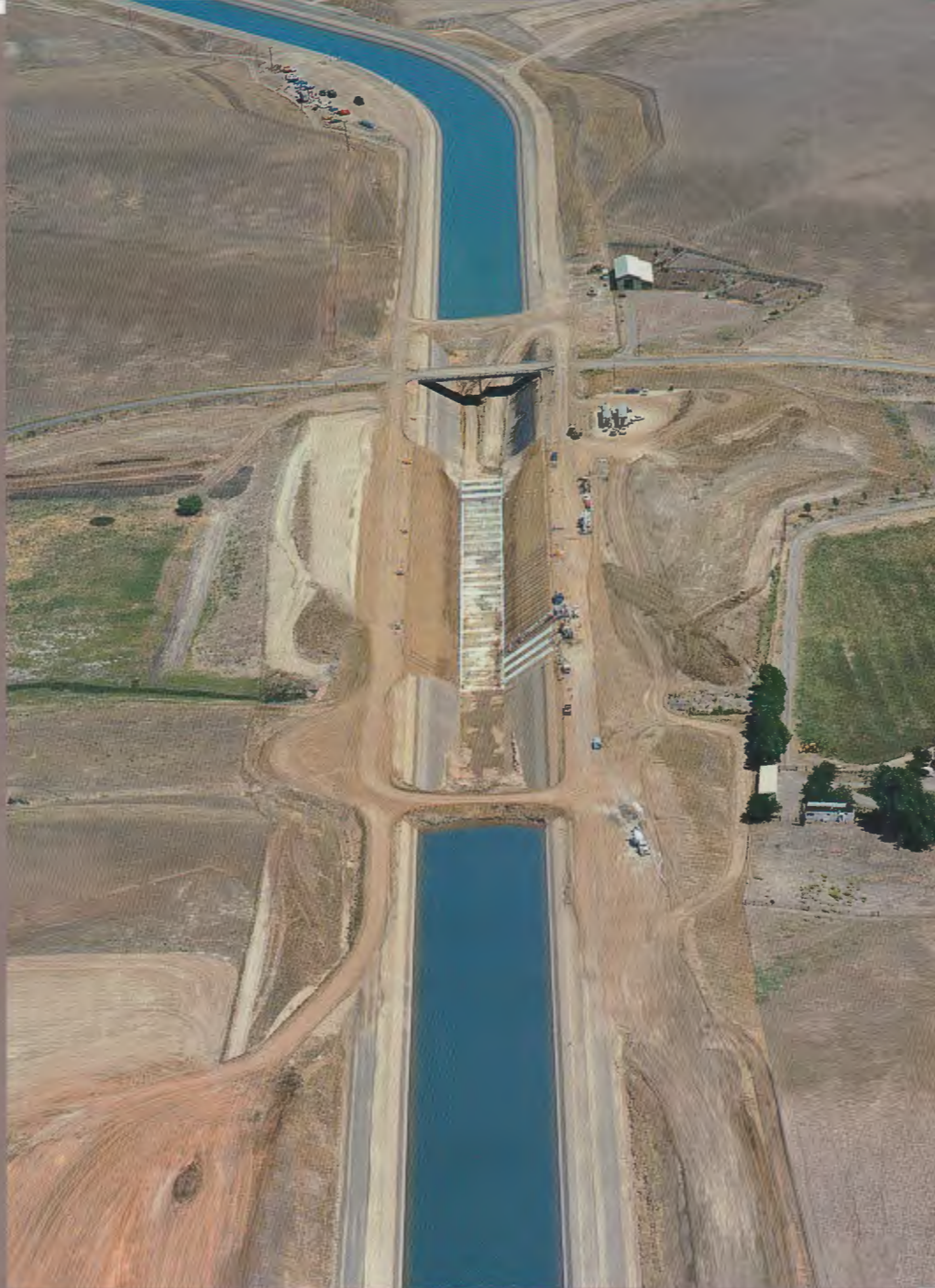
Repair at mile 56 was a planned outage in 1990. Canal lining is underway (above).
