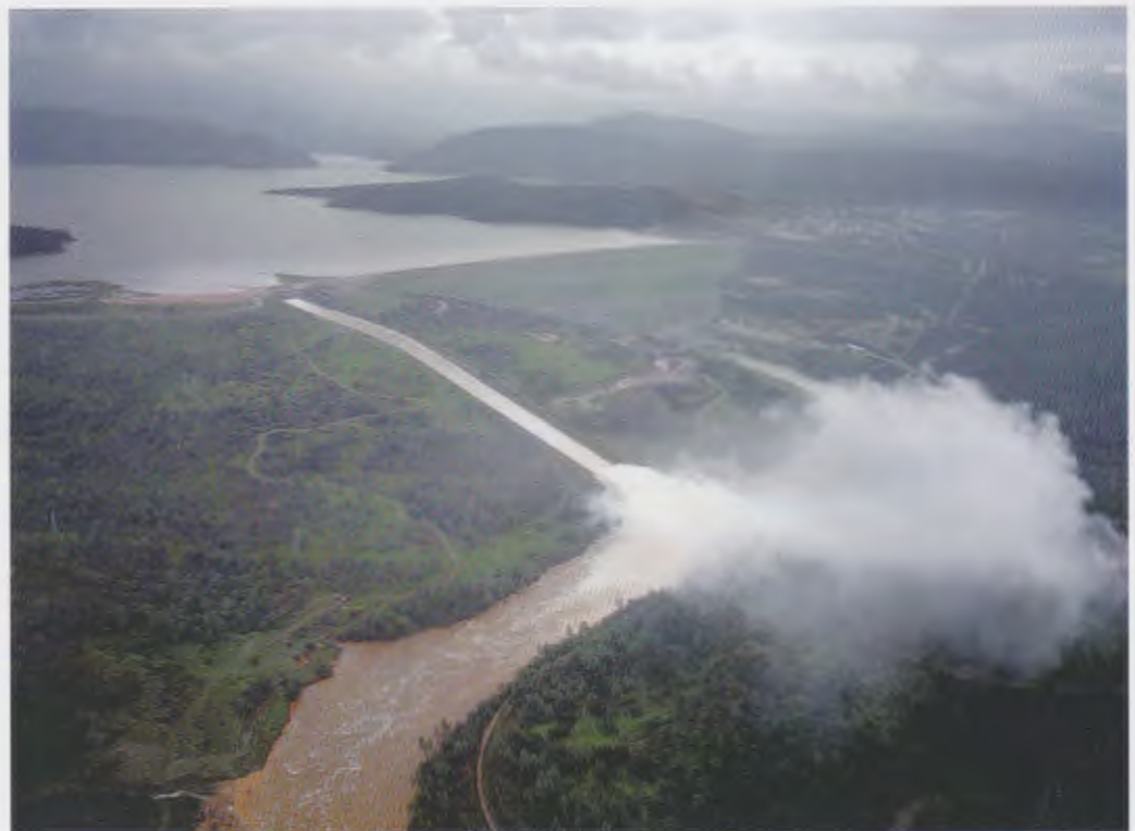
Water being released down Oroville Dam spillway.
