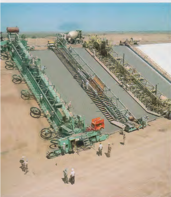
Paving train for the California Aqueduct.
