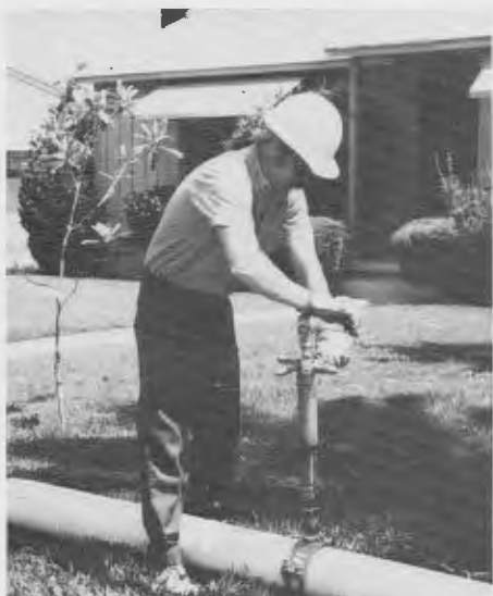
Mesa Consolidated crewman taps into pipe on repair project.
