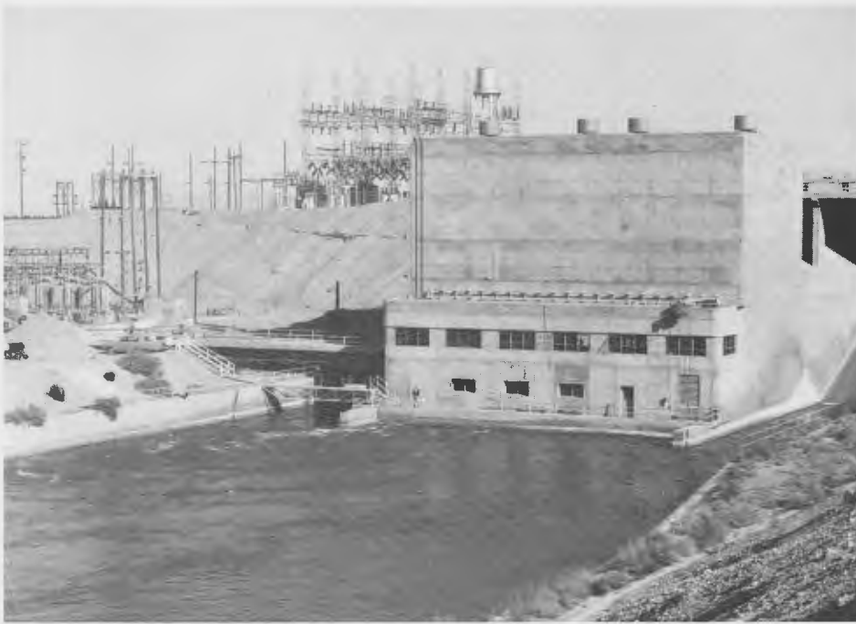
An Imperial Irrigation District hydroelectric generation plant on the All-American Canal is shown above. It is one of five such facilities.
