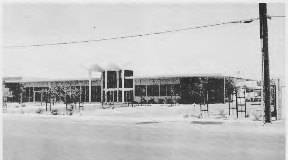
Above is headquarters building for Imperial Irrigation District, providing the base from which staff serves the Imperial Valley.
