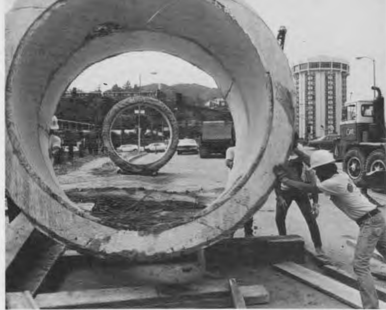
Metropolitan Water District of Southern California crew prepares pipe for installation.
