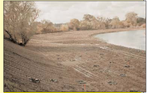
The filled and planted pool left — now riparian floodplain and forest — and new channel right. Courtesy Turlock Irrigation District
