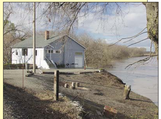
House at the top of failing "J" levee near Hamilton City. City residents and local government are getting a taste of the new approach to restoration along the Sacramento River, working with the Army Corps, the Department of Water Resources, the Forum, the Nature Conservancy, and others to replace an old and failing levee that can no longer protect the city from floods with a setback levee that will give the river more meander room. The project design meets both ecosystem and flood control objectives, and puts restoration dollars to work to protect the homes and livelihoods of local residents and farmers.
