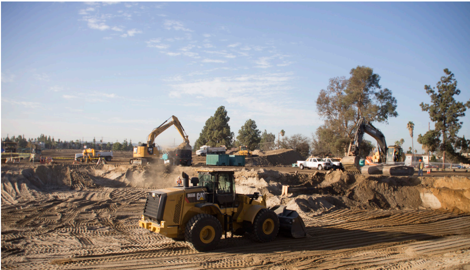
NHW Well Field Treatment Facilities Construction Begins (2017)
