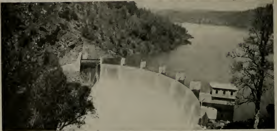
Present Melones Dam Completed in 1926
