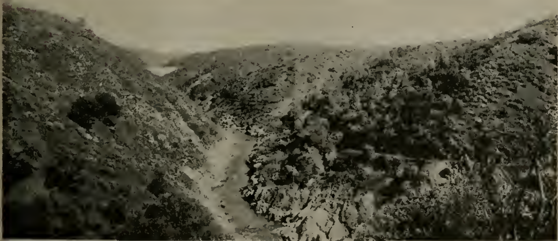
Site of Proposed Dam Below Existing Structure
