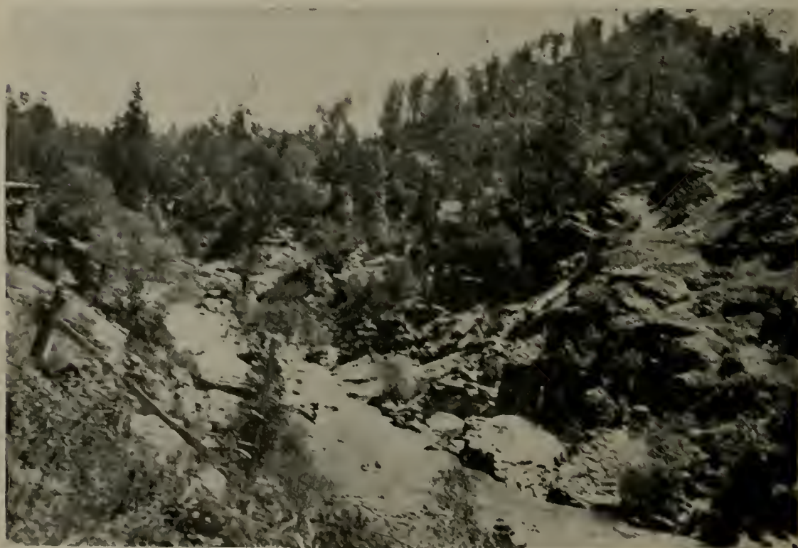
WINDY GAP DAM SITE ON FRESNO RIVER
