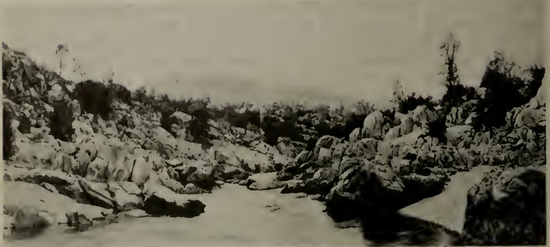
Site of Main Isabella Dam
