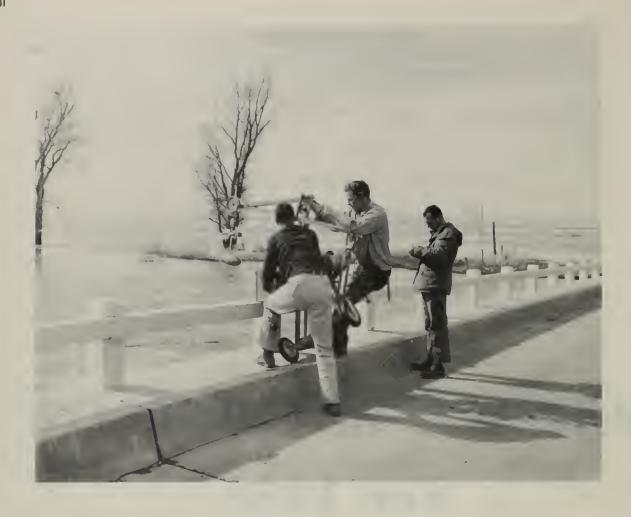
DISCHARGE MEASUREMENT OF YOLO BYPASS NEAR WOODLAND
