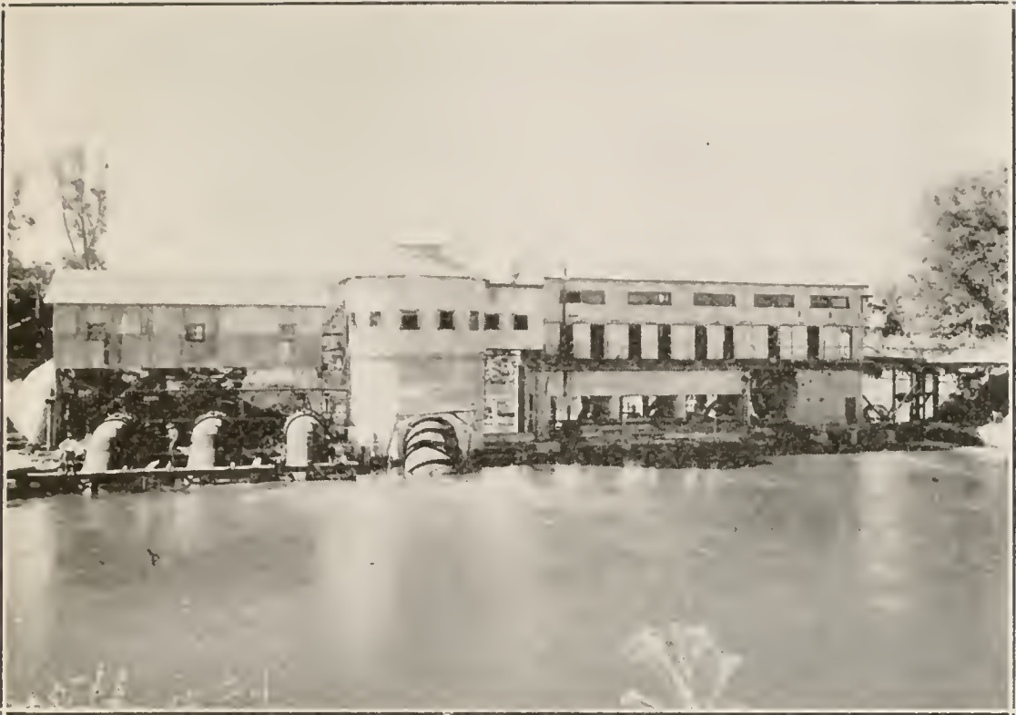
FIG. 1. Pumping plant furnishing 1500 cubic feet of water per second to Central Canal, Glenn-Colusa Irrigation District.
