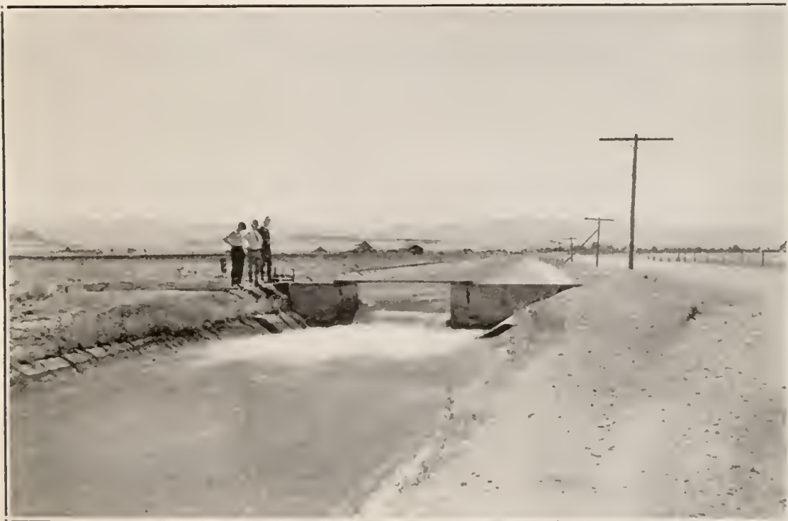
FIG. 2. A concrete-lined irrigation canal on the Orland Project of the United States Reclamation Bureau.
