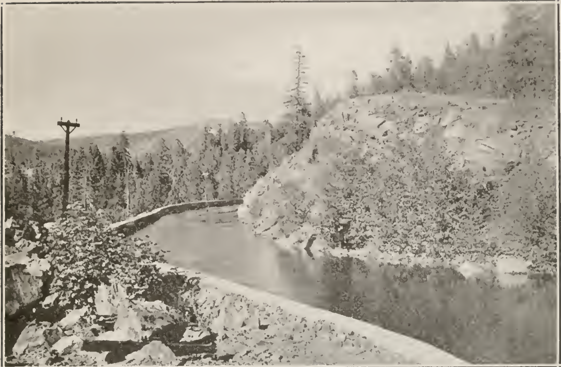
FIG. 1. A combined power and irrigation canal in the Sierra Nevada above Sacramento Valley.
