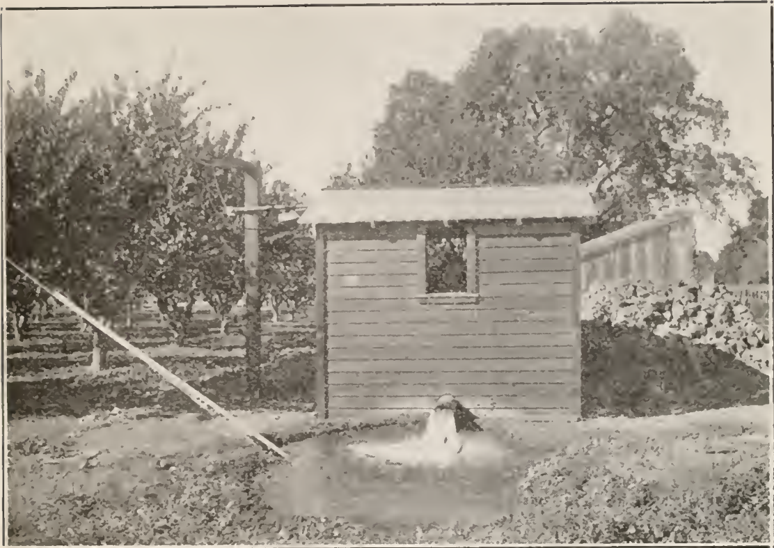
FIG. 1. A typical small irrigation pumping plant in Santa Clara Valley.
