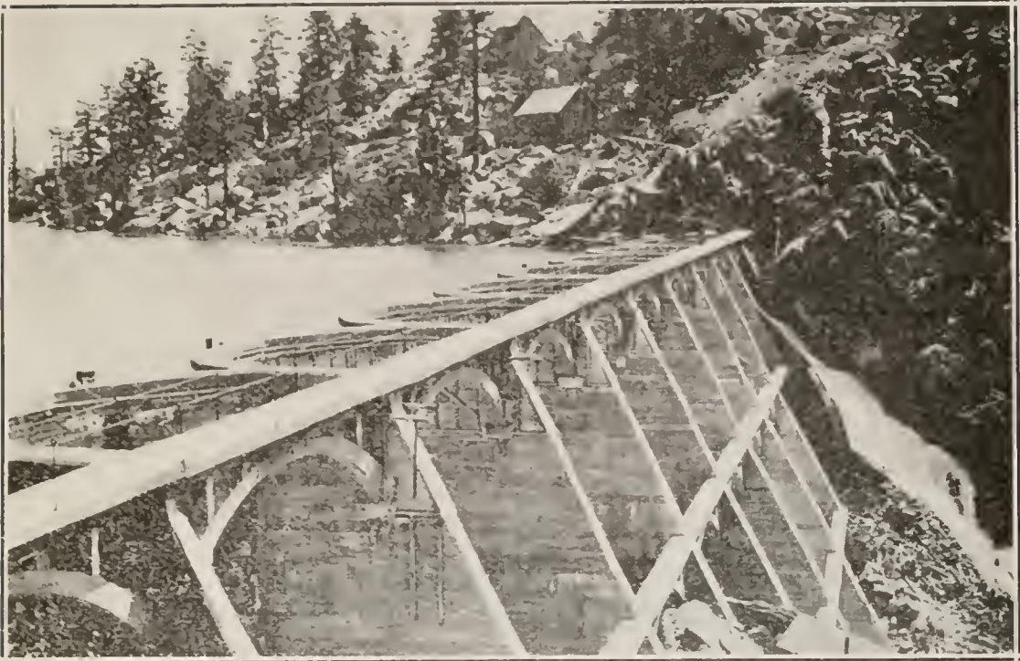
FIG. 1. Bear Valley Dam in the San Bernardino Mountains, storing irrigation water for important citrus areas in San Bernardino County.
