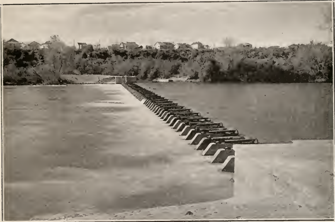
FIG. 1. Dam across Sacramento River at head of Anderson-Cottonwood Irrigation District.
