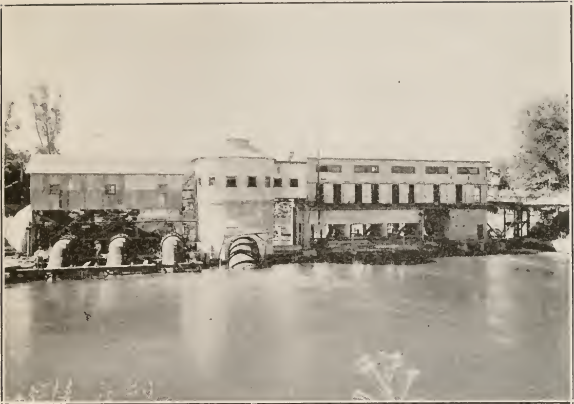
FIG. 1. Pumping plant furnishing 1500 cubic feet of water per second to Central Canal, Glenn-Colusa Irrigation District.
