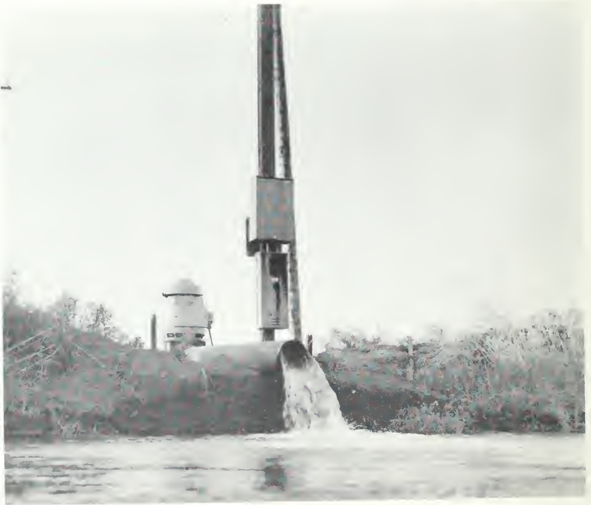
Deep Well and Turbine Pump Installation in Sutter-Yuba Area
