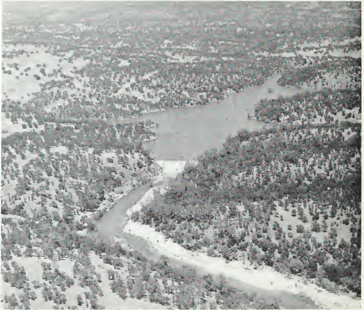
Existing Camp Far West Dam and Reservoir
