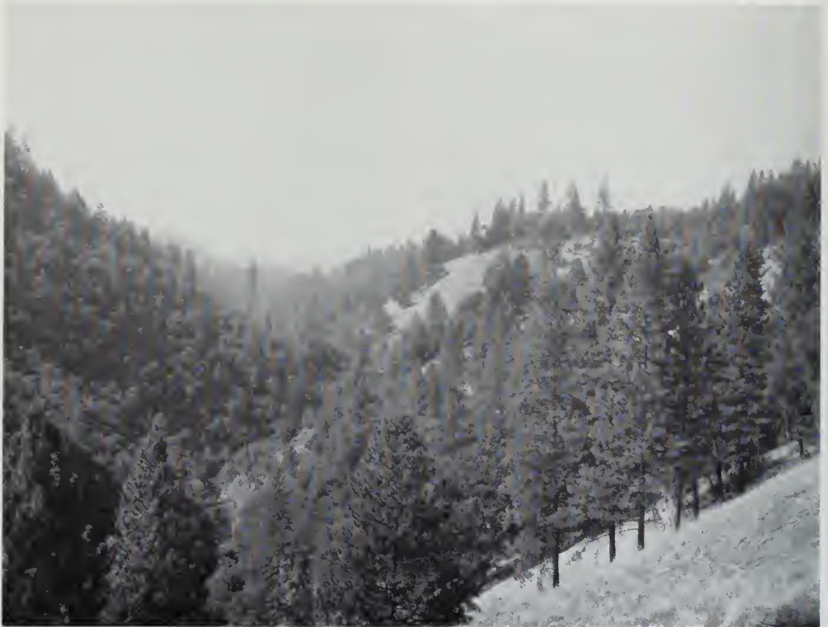
Railroad Flat Dam Site, South Fork of Mokelumne River
