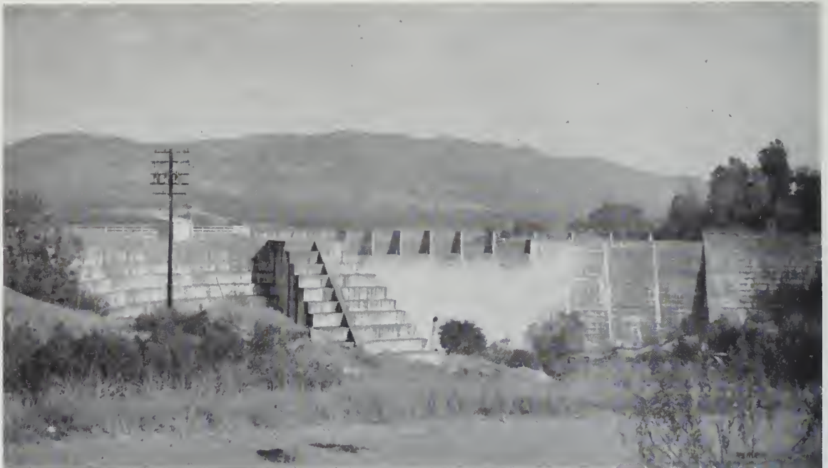
Hogan Dam on Calaveras River
