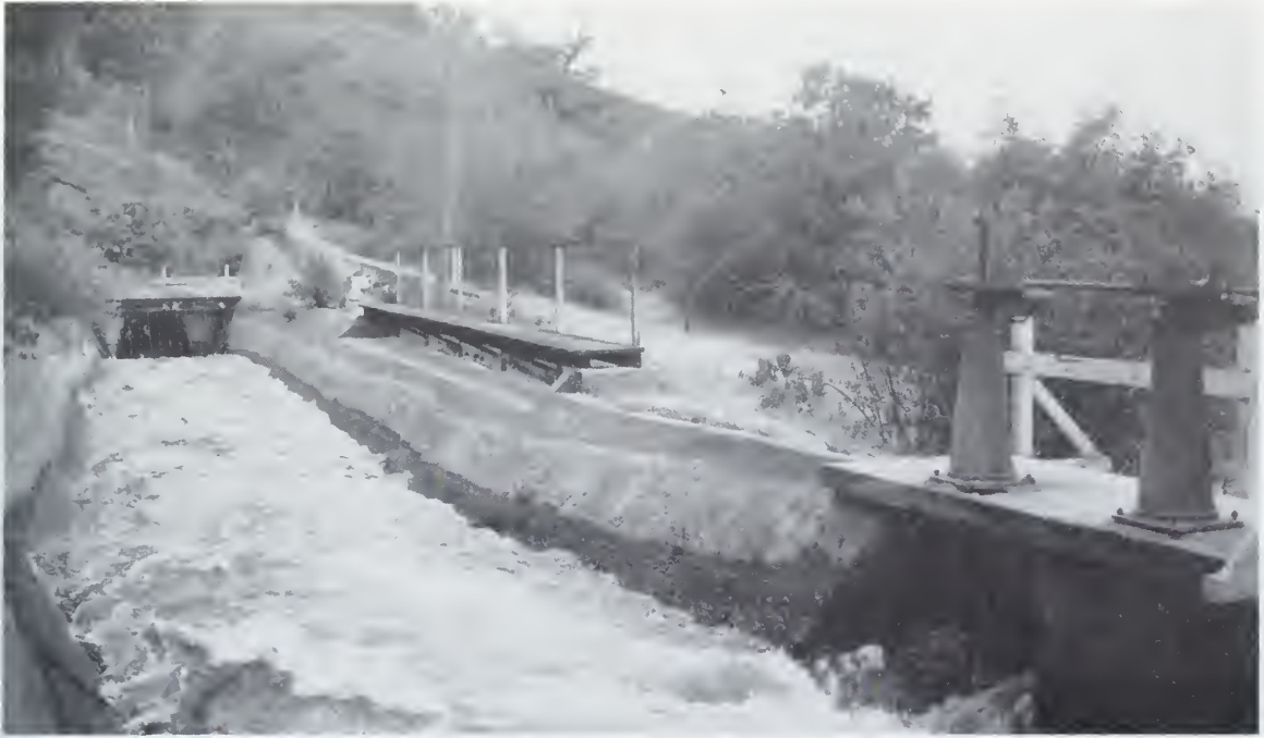
South Canal at Tunnel II
