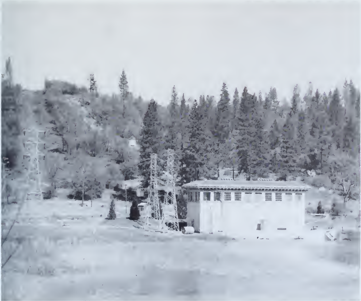
Halsey Power House
