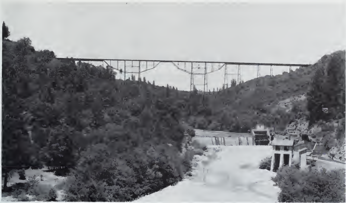
Rollins Dam Site and Bear River Canal Intake
