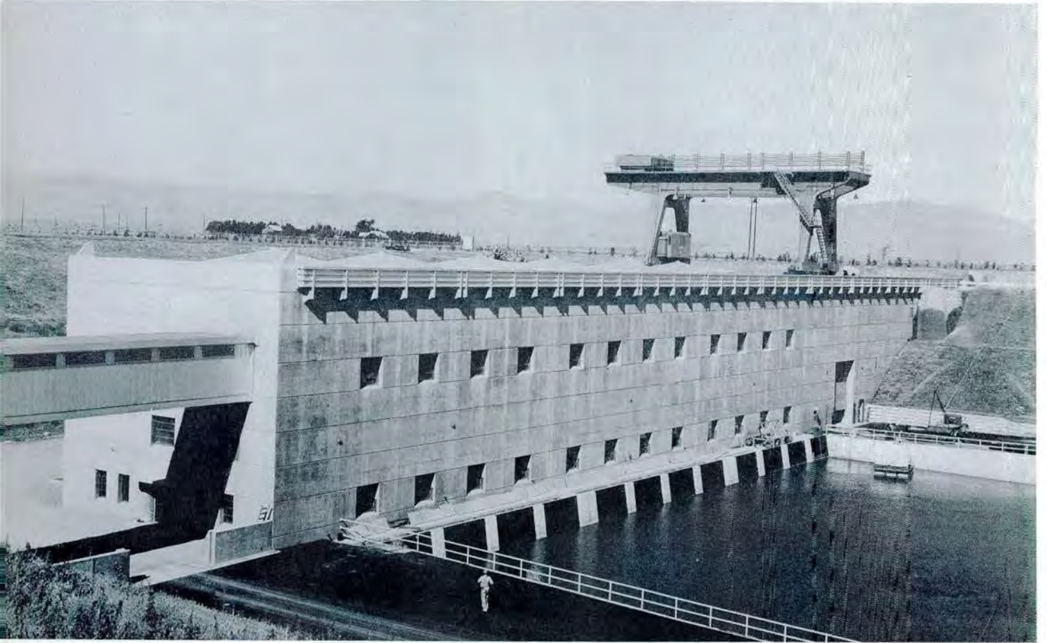
Delta Division—Constructed Features of the California Aqueduct System. Delta Cross-Channel Headworks on the Sacramento River and the Tracy Pumping Plant on Old River
