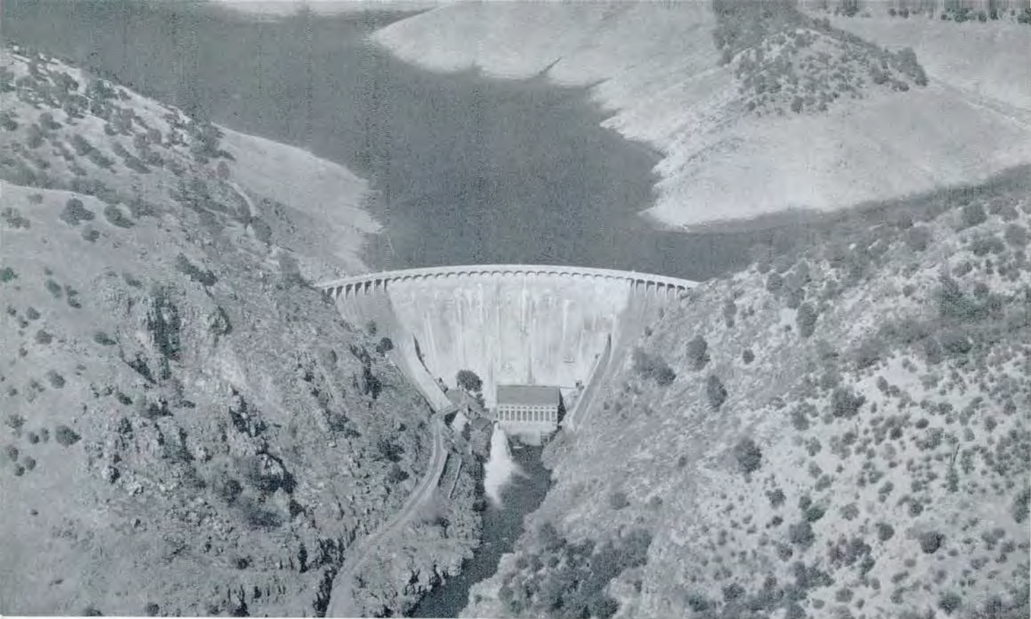
Exchequer Dam on Merced River
