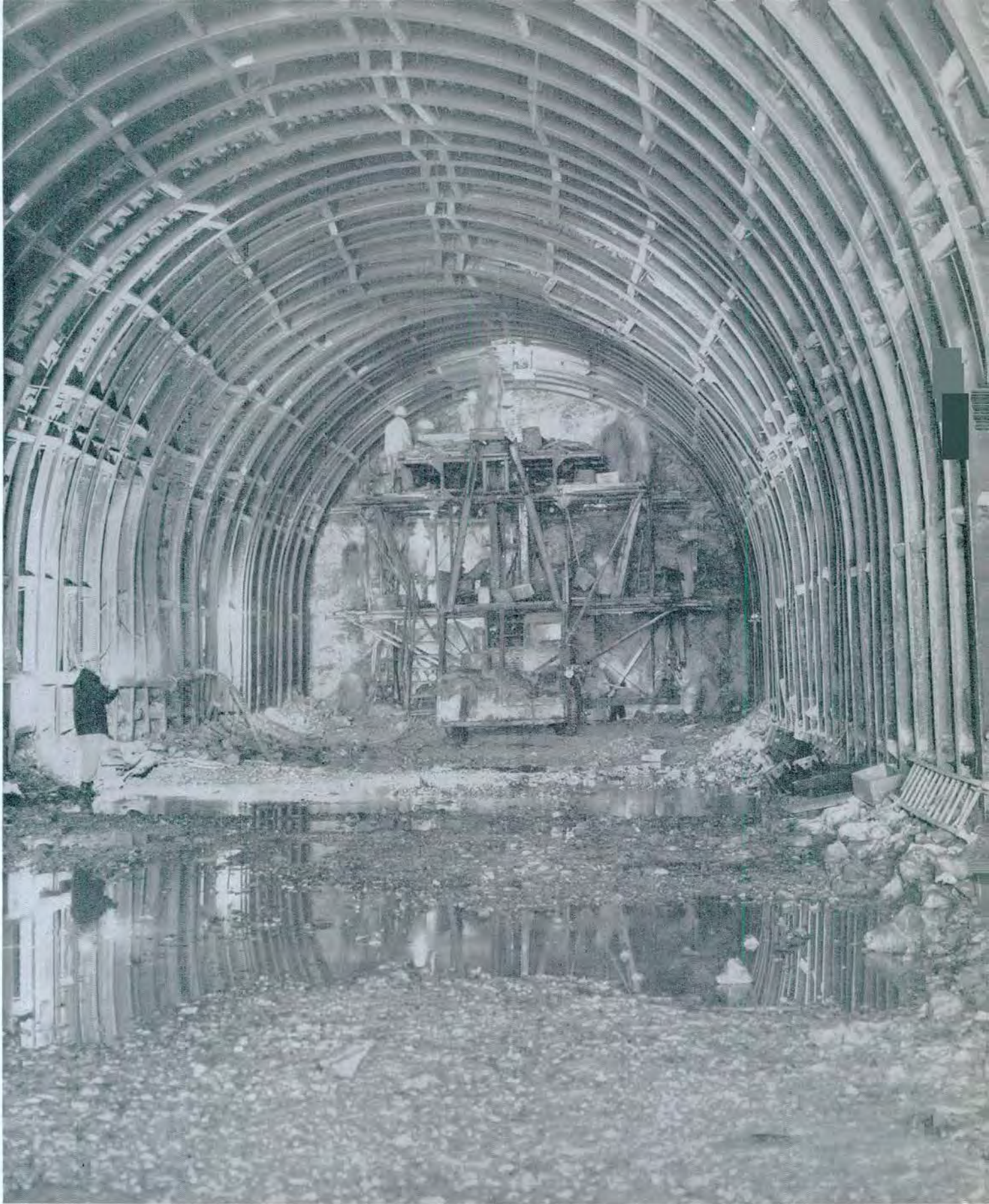
Klamath-Trinity Division—Head of Tower House Tunnel of the Trinity Diversion Project
